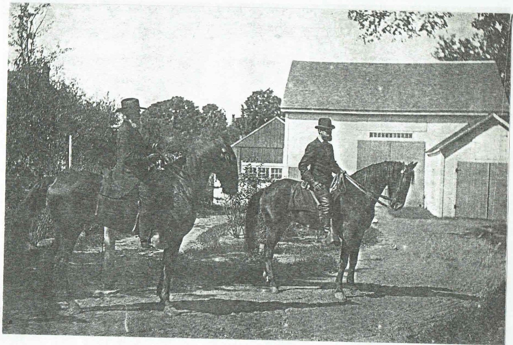
"Henry Shepherd on 'Mr. Fox' and Thomas Munroe on 'Brer' Rabbit' in homestead yard (66 Bridge Street) Return from Hatfield trip-September 26, 1898." Note rose garden at center of turn-around, vanished outbuildings at side of barn, vanished hitching post behind Mr. Fox.
