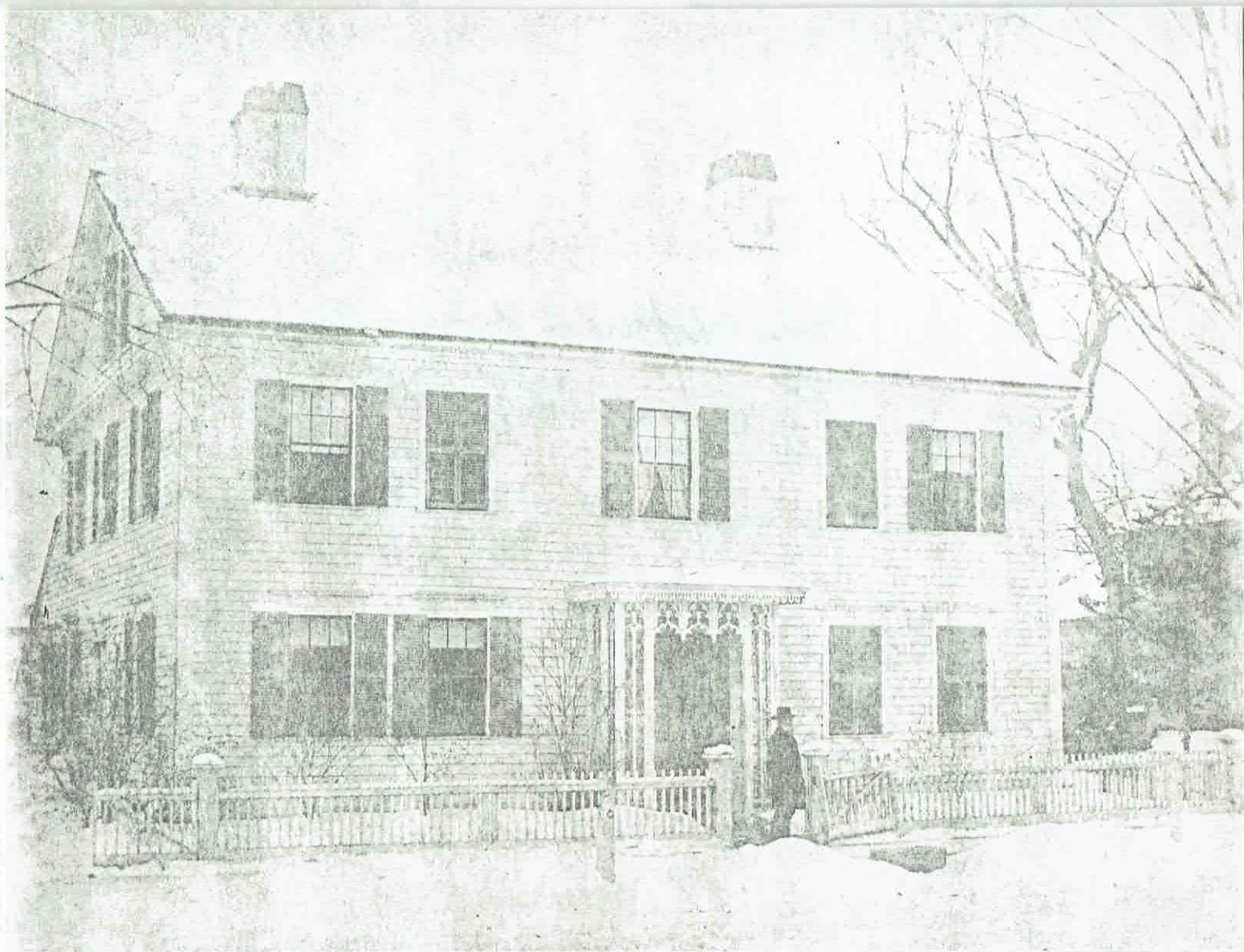
Photograph circa 1895 of Shepherd House. Picket fencing and gates enclose the property at the sidewalk line. Posts are at gates and ends, while intermediate support is provided by stone supports behind the fence line. Note also the lack of the side porch, deciduous plantings at the front and side, stone hitching posts and stairs at the street edge. [Henry Shepherd in doorway].
