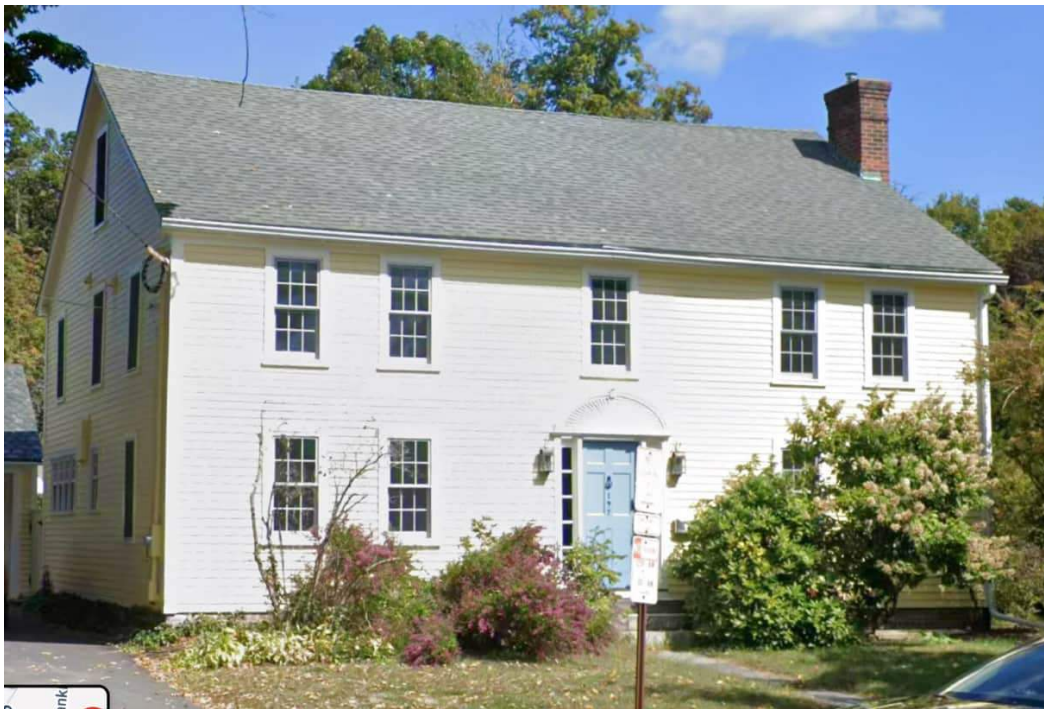
Figure 38: Ebenezer Clark House 1730 c. 197 Elm Street, Northampton, MA. (Image courtesy of Google Maps.)
