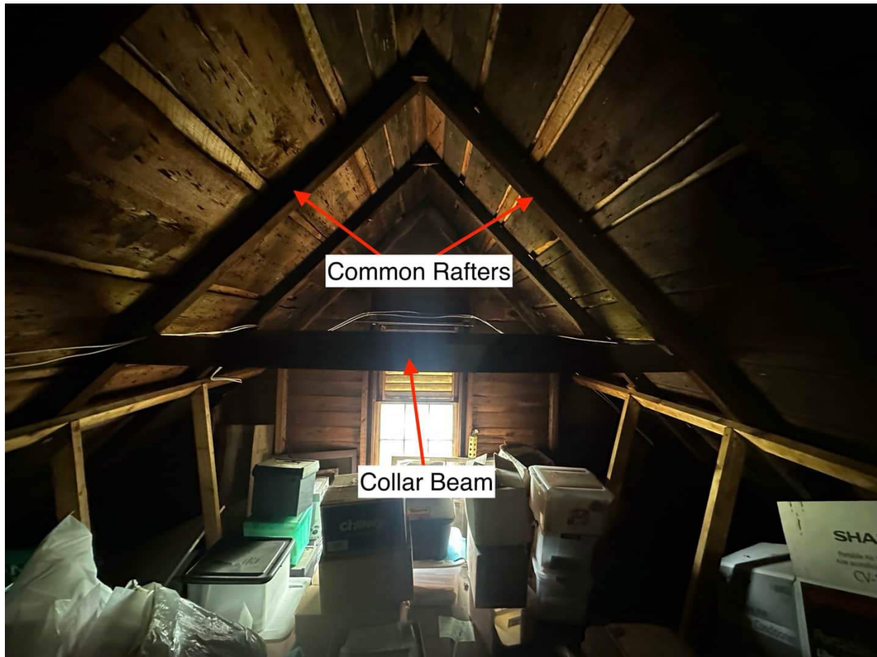
Figure 29: Common rafter and collar roof system of the John Moore house 1666 c. in South Windsor, CT. (Photograph by Nevan Carling.)
