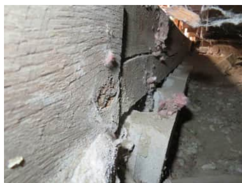
Condition of south wall of west block. Top: After trim removal; Bottom Left: Replacement sill condition above grade; Bottom Right: View of shifting CMU foundation and sill.
