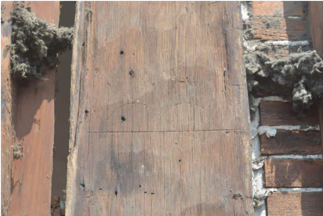
Figure 9: Two-foot mark on the post of the 1722 d. Riley/Adams house formerly in Wethersfield, CT. (Photograph by Nevan Carling.)
