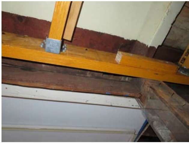
Top: Ledger at south side of infill, overview and east end (not fastened) respectively; Bottom Left: Central portion of south ledger; Bottom Right: Notch in joist from former waste pipe
