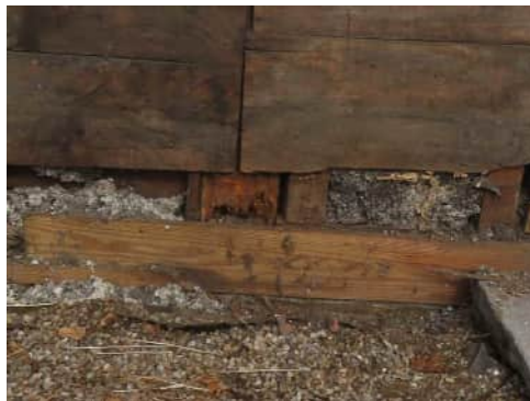
Condition of south wall of west block. Top: After trim removal; Bottom Left: Replacement sill condition above grade; Bottom Right: View of shifting CMU foundation and sill.
