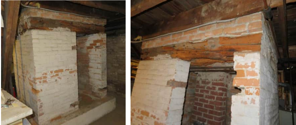
Kitchen Ell chimney mass base from the north
