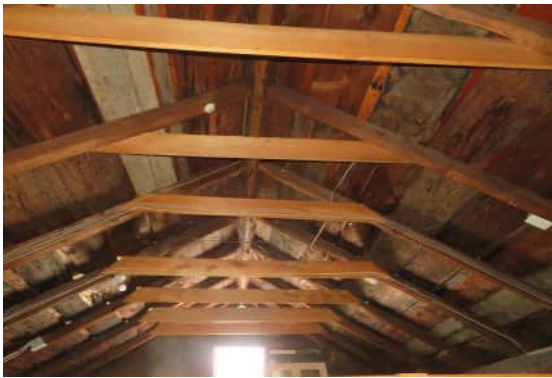
Original House roof framing showing 5-sided ridge pole; common rafters and central purlin
