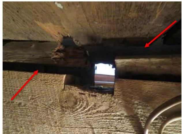
Directly below east wall panel from east showing gaps in 2 different views
