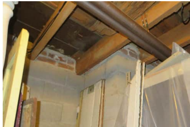
West (original rubble stone) and east (1981-82 CMU underpinning) side of main chimney mass base respectively
