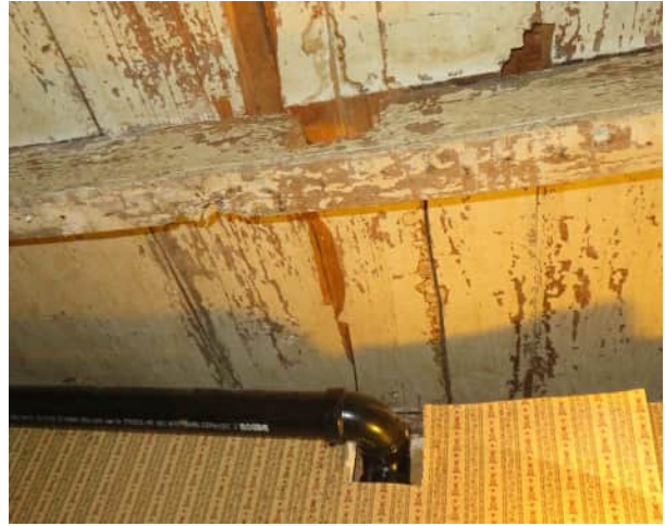
Top: Ledger at south side of infill, overview and east end (not fastened) respectively; Bottom Left: Central portion of south ledger; Bottom Right: Notch in joist from former waste pipe
