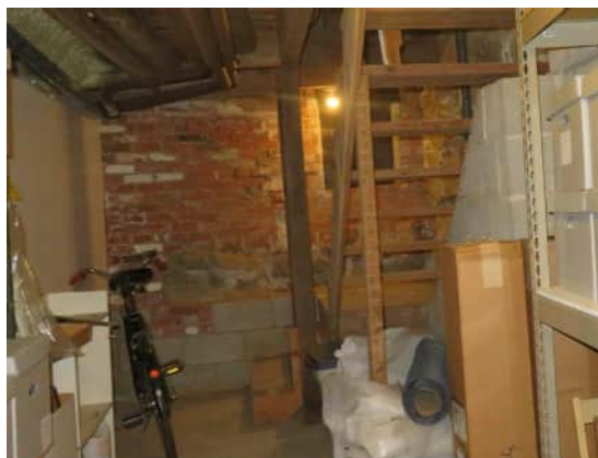
Left: Brick infill wall between west (higher / original) basement and east lower basement, note CMU underpinning below brick and along south wall of the chimney mass; Right: Excerpt from 1979 Rexford drawing showing narrow basement below front vestibule prior to underpinning and constructing full east basement in 1981/82.
