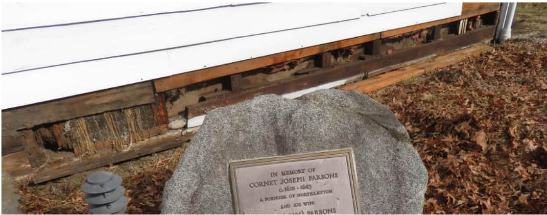
Exposed south sill, east block overall
