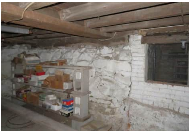
West (original rubble stone) and east (1981-82 CMU underpinning) side of main chimney mass base respectively
