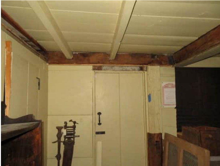
Second floor joists framing into the north wall plate with diminished bearing visible after removal of trim board.
