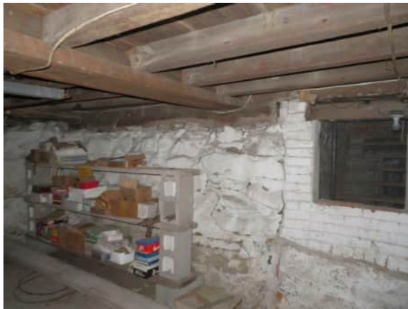
West wall of chimney base showing bulge and compressed chimney girt
