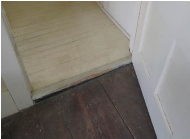
Left: Second floor door threshold above stair infill showing floor deflection; Right: Overall view of lean-to framing showing sag
