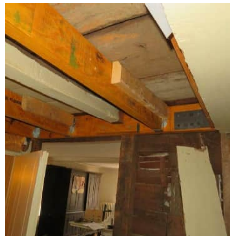
Infill framing at former stair opening looking north and south respectively
