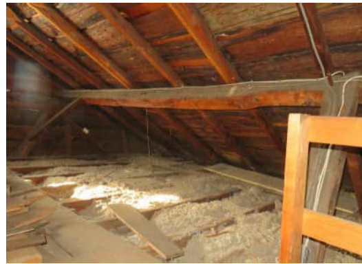
Original House roof framing showing 5-sided ridge pole; common rafters and central purlin
