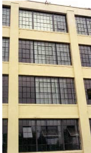
Fig. 15. Original steel windows were retained and made operable during the rehabilitation of this historic mill complex. Insulated sliding windows were added on the interior to improve energy efficiency.
