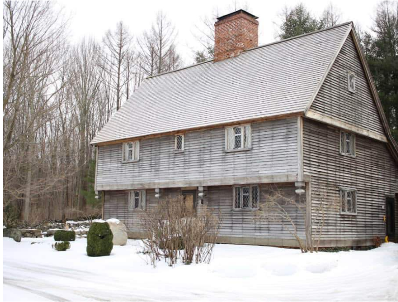
Figure 6: The 1700 c. William Hill House formerly located in East Hartford, CT with a framed jetty. (Photograph by Nevan Carling.)
