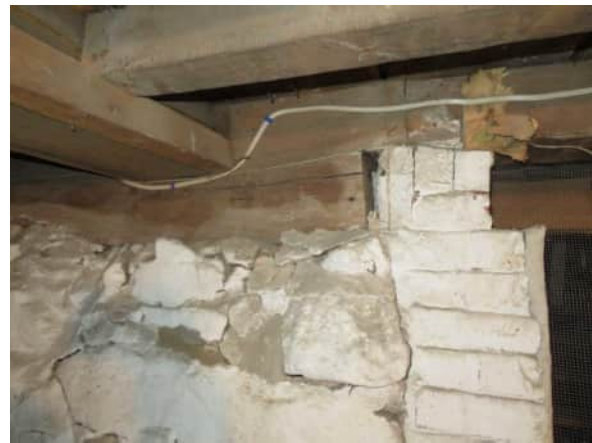
West wall of chimney base showing bulge and compressed chimney girt
