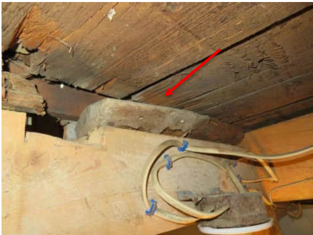
Directly below east wall panel from east showing gaps in 2 different views
