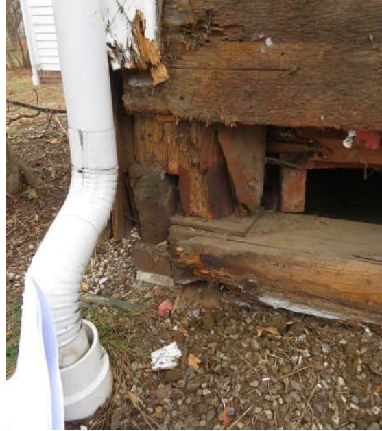
Left: Southwest corner inside basement showing salts from water ingress and dark staining suggestive of mold (note CMU bulkhead infill); Right: Southwest corner on exterior showing deteriorated sill and post base.
