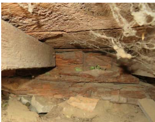
View of decayed inner sill and suspended short joist end (not bearing on outer sill), respectively.
