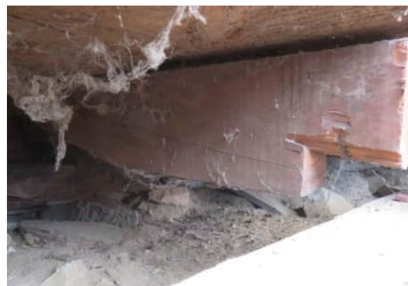
View of decayed inner sill and suspended short joist end (not bearing on outer sill), respectively.
