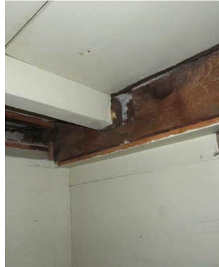
Second floor joists framing into the north wall plate with diminished bearing visible after removal of trim board.
