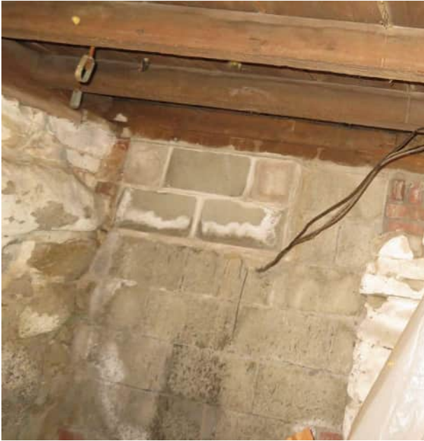
Left: Southwest corner inside basement showing salts from water ingress and dark staining suggestive of mold (note CMU bulkhead infill); Right: Southwest corner on exterior showing deteriorated sill and post base.
