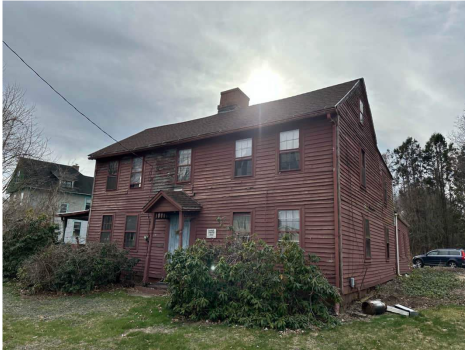
Figure 35: Samuel Porter house 1730 c. East Windsor, CT –saltbox later addition. (Photograph by Nevan Carling.)
