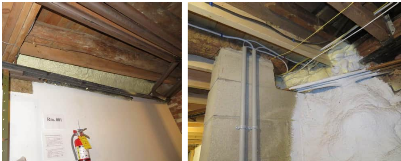
Multiple generations of spray foam insulation apparent in the basement, particularly along the perimeters of the building
