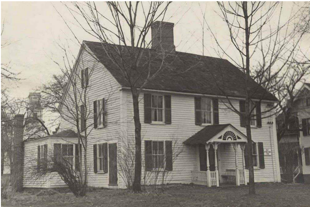
Figure 36: Return Strong house 1720-40 c. Windsor, CT. (Photograph courtesy of the Windsor Historical Society.)
