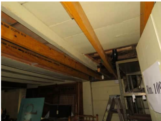
Infill framing at former stair opening looking north and south respectively
