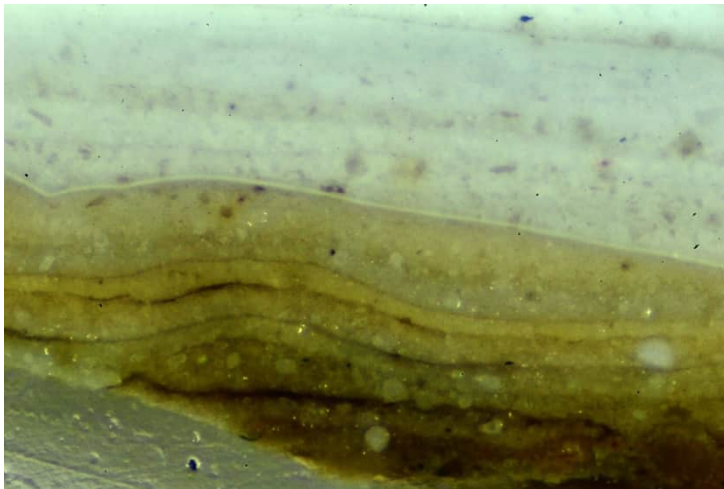
067 South wall wainscot at west end
