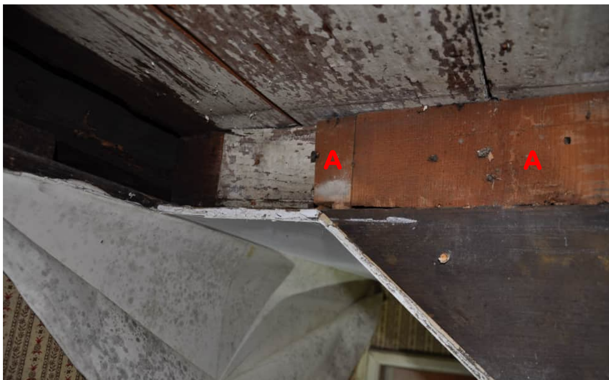
Figure 31. View of the east side of the remnants of vertical boards A which formed the east wall of the Phase 3 staircase. The vertical boards forming this wall were nailed to the east side of the joist with Type 2 machine-cut nails. Note that the unpainted vertical boards were applied over whitewash on the joists and ceiling boards. The lath and plaster ceiling were created after the staircase was in place, made evident by the unpainted section of the vertical boards above the level of the plaster ceiling. A nailer for the lath was applied over the vertical boards at joist level (removed at the time of this photograph). This nailer was a reused element. It was painted with a yellow/ochre distemper paint, the first-generation paint on the sheathing, providing further evidence that the staircase was likely erected during Phase 3 rather than Phase 2. The plaster ceiling in this space was removed in the late 20 th century when a bathroom was created in this space, and several of the vertical boards were sawn off at the level of the joists to create a passageway into the new bathroom. (Photograph by Myron O. Stachiw, 2024.)
