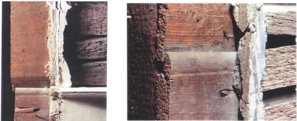
Figure 9. Detail views of the Phase 1 sheathing of the interior walls of the hall or kitchen (Rm 102). Phase 2 lath and plaster and wainscot were applied in the early 19 th century over the Phase 1 sheathing. The Phase 1 sheathing exposed in these photographs was covered by an architrave surrounding a doorway to the rear lean-to. The mill-sawn boards, which measured between 8 and 12 inches in width, were planed smooth on one face and finished with a feathered lower edge and molded top edge. The feathered lower edge of the upper board fit behind the molded upper edge of the board beneath it. (Photographs 102-5 and 102-6 from Clancey and Leeke, 1992.)
