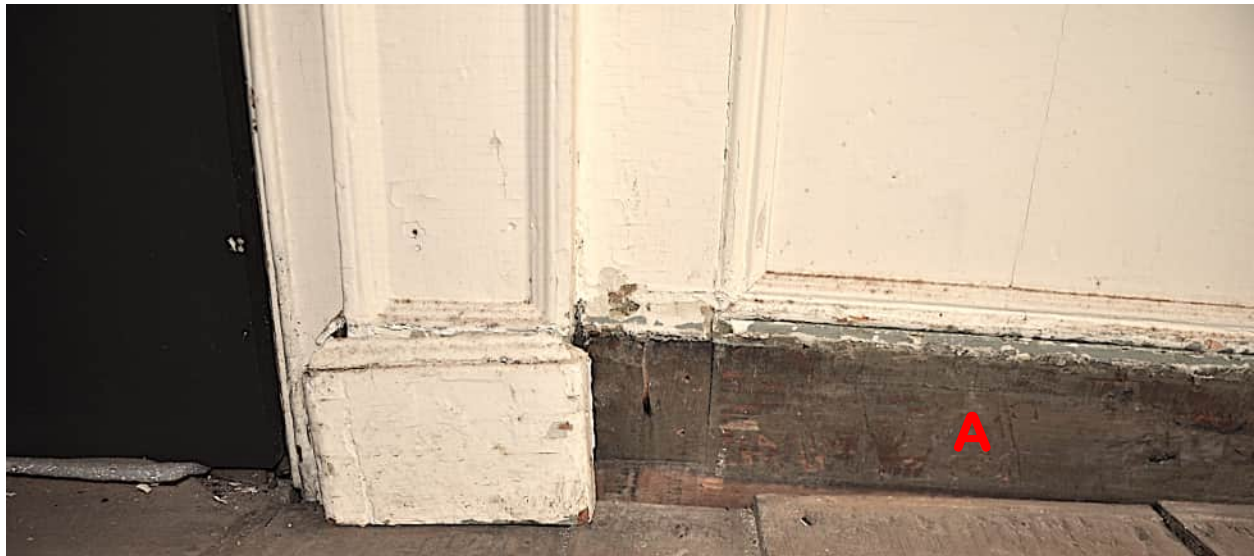
Figure 76. Detail view of the lower edge of the chimney breast paneling in Rm 112 after removal of the applied Phase 4 baseboard. A indicates the Phase 2 dark brown painted mopboard on the lower end of the rails and stiles of the paneled wall. The same painted mopboard was also found on the wainscot on the other walls in Rm 112. (Photograph by Myron O. Stachiw, 2024.)
