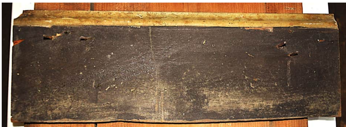
Figure 77. Reused polychrome baseboard fragment found in Rm 102. This same combination of light and dark paints on the baseboard was found in several rooms in the house applied over the earlier painted mopboards. (Photograph by Myron O. Stachiw, 2024.)
