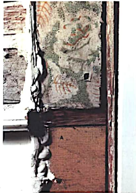
Figure 49. The second-generation wallpaper on the walls of the hall/kitchen was preserved only under the west architrave of the doorway to Rm 104. It is likely that this wallpaper was applied as a complement to the yellow tan paint visible on the wainscot in the above image 102-17, as both the wallpaper and the tan-colored wainscot were covered by the door architrave. This wallpaper was applied late in Phase 2 or during Phase 3, as some of the woodwork in this room has shown as much as four layers of the yellow tan paint. The color swatch provides a close approximation of the original color of the yellow tan paint on the wainscot and other woodwork in this room. This doorway to Room 104 was created during the Phase 4 improvements (Photograph from Clancey and Leeke, 1992.)
