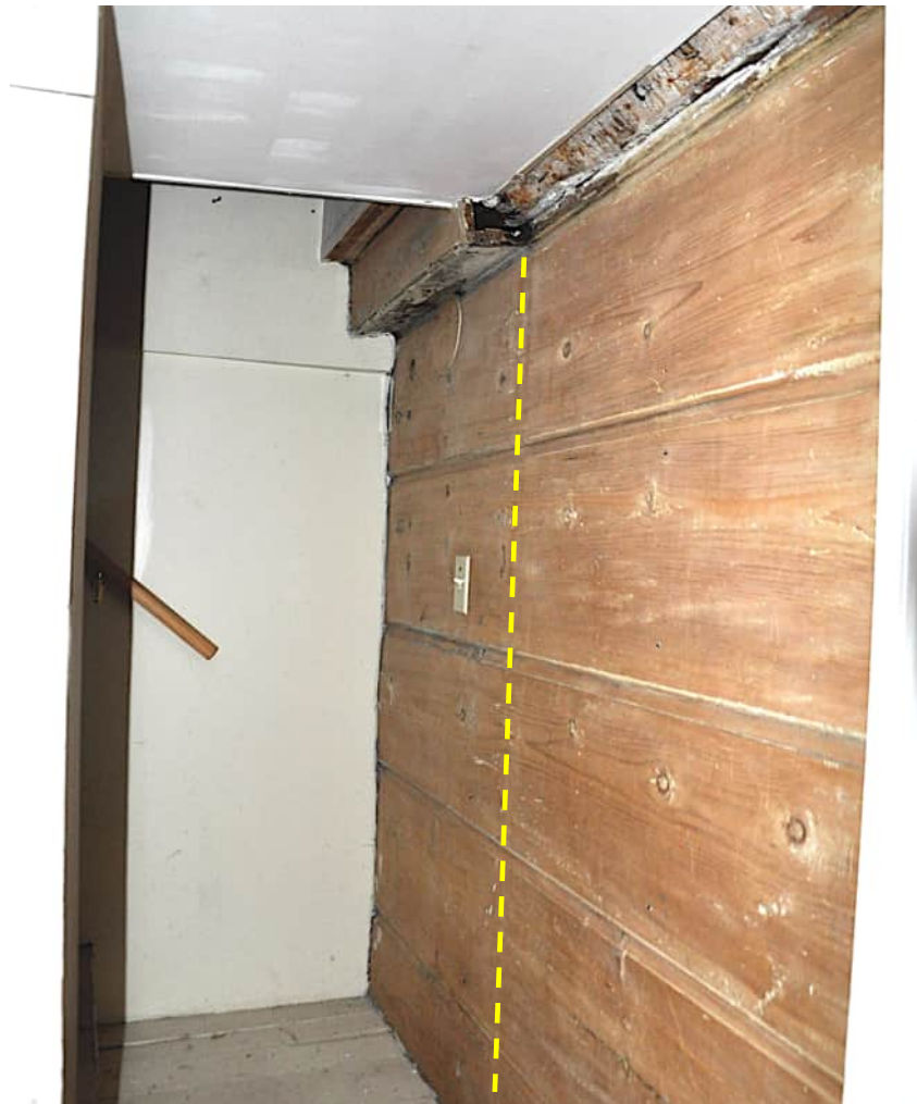
Figure 29. View of the horizontal, molded board sheathing on the north wall of Rm 104. These sheathing boards are continuous past the staircase and wall at left into Rm 109, suggesting that the rear staircase to the second floor and the room partitions across the rear lean-to were created after the walls were fully sheathed. The yellow dashed line indicates the location of a vertical scribe line on the surface of the sheathing boards which coincides with the location of the east wall of the original Phase 3- and present staircase. (Photograph by Myron O. Stachiw, 2024.)
