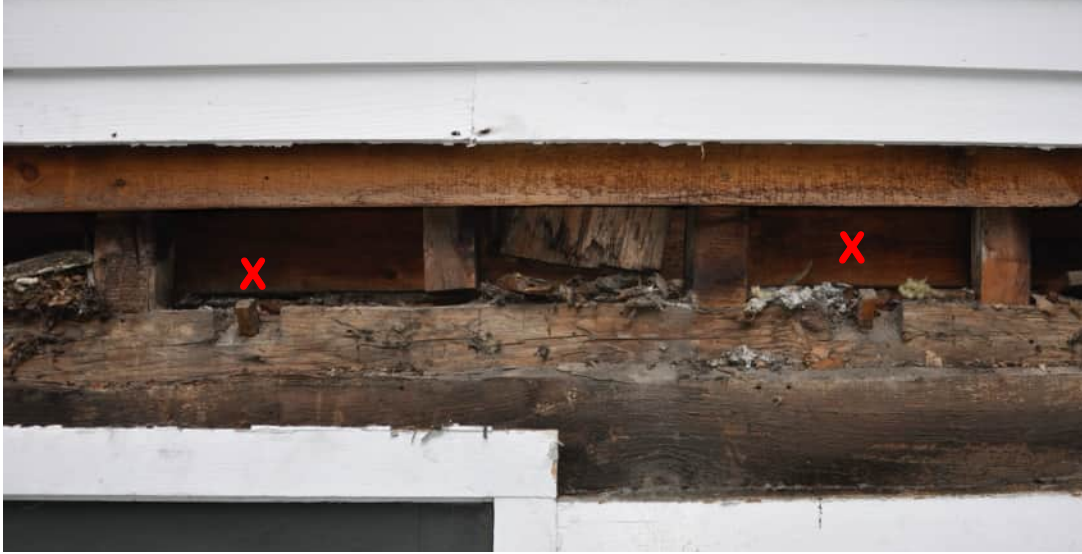
Figure 27. View of the north- or rear plate of the Phase 2 lean-to. Two step-mortises for the rafter feet of the Phase 2 lean-to roof rafters are indicated by X. Note the pegs which fastened the lower end of the rafters to the plate still in place in these mortises. The lower ends of a post and several studs are visible above the plate forming the south wall of the second-story rooms created when the Phase 2 rear lean-to was raised to two full stories in 1816 (Phase 3). (Photograph by Myron O. Stachiw, 2024.)
