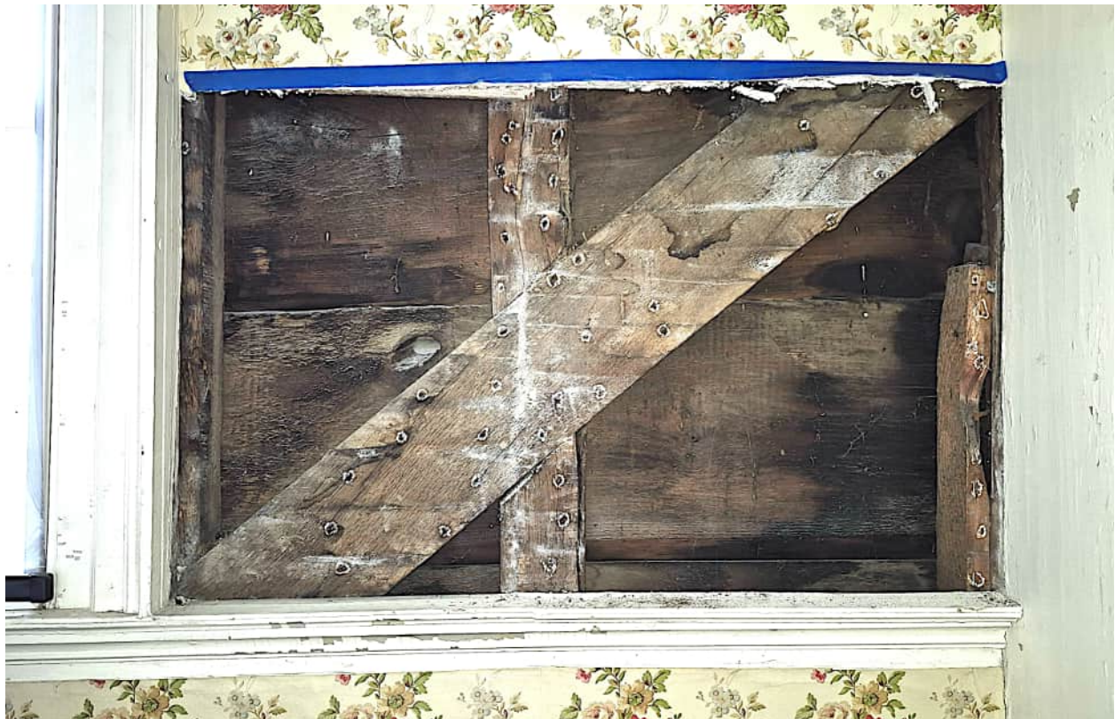
Figure 22. View of the 2025 excavation through the south wall of Rm 210. The early 19 th century plaster and sawn- and split lath were removed, and the nail holes left by the early machine-cut nails which fastened the lath were marked. No extraneous nail holes from earlier finishes were discovered, supporting the conclusion reached by the investigators during the 1992 study that the walls of the second-floor rooms remained unfinished through the 18 th century. Investigation of the ceiling in this room from the attic revealed that the sawn- and split lath applied to the ceiling in this room were not nailed to the underside of the attic floor joists, but to nailers suspended several inches below the joists. This allowed examination of the undersides of the attic floor joists; no nail holes from any earlier lath or board sheathing were discovered, confirming that the two second-floor rooms did not receive lath and plaster ceilings until the early 19 th century, probably at the same time that the walls of these rooms were lathed and plastered. (Photograph by Myron O. Stachiw 2025.)
