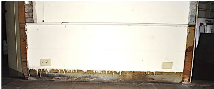
Figure 42. View of the Phase 2 wainscot on the north wall of the hall/kitchen (Rm 102). When first applied the wainscot was decorated with a red-painted mopboard (See Figure 45.) During Phase 3 or 4 a molded baseboard was applied over the painted mopboard. The doorway at left opens onto Rm 109 of the Phase 2 rear lean-to in the same location as the doorway into the Phase 1 lean-to. The Phase 1 horizontal boards on the interior walls of the hall/kitchen are visible after removal of the Phase 4 door architrave on the left doorway to Rm 109. The existing architrave on this doorway was installed during Phase 4 to match the architrave on the new doorway on the right created during Phase 4 after the east addition was constructed. Note that the architrave on the right-hand doorway was applied over the painted Phase 2 wainscoting. (Photograph by Myron O. Stachiw, 2024.)
