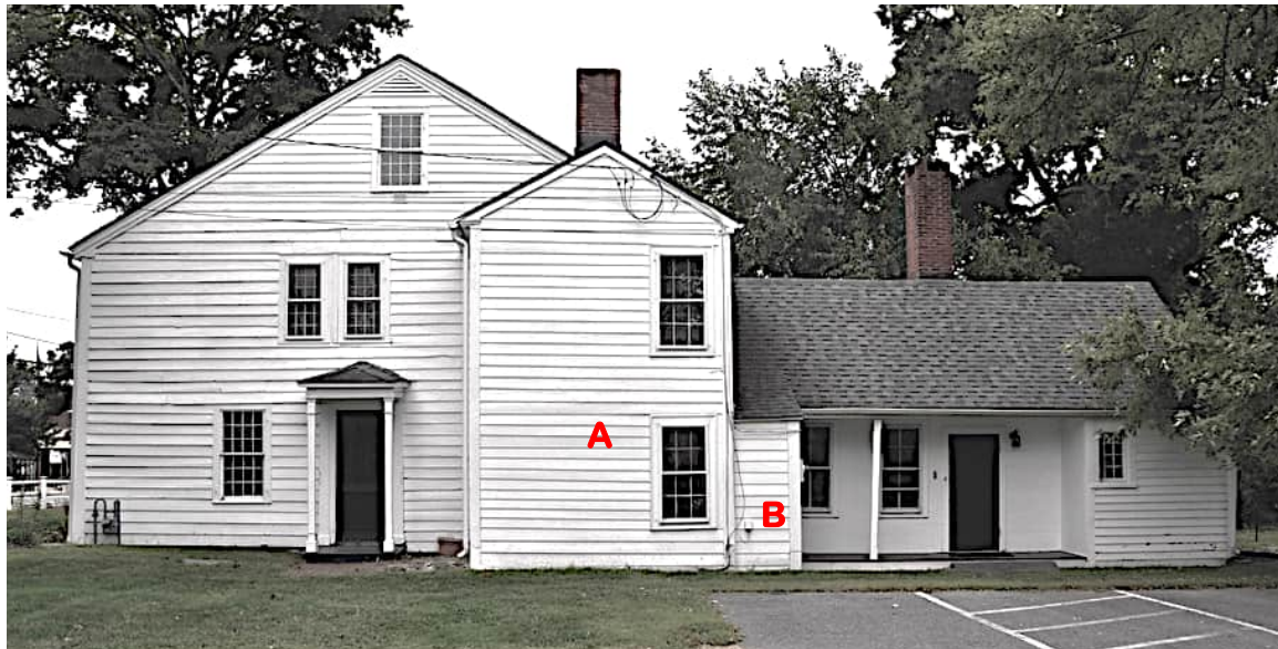
Figure 70. Above - View of the east elevation of the Parsons House, looking to the southwest. The Phase 4 two-story east wing is in the center (marked A ), and the surviving section of the Phase 5 rear kitchen ell is at right. B represents an added cupboard on the north wall of Rm 104.
