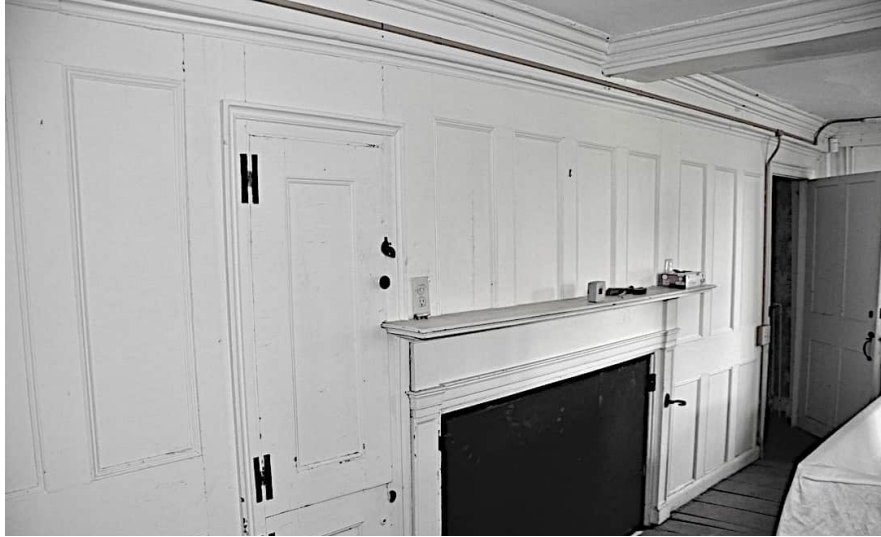
Figure 51. View of the new Phase 2 paneled chimney breast wall applied to the east wall of the parlor. The present mantelpiece was applied during Phase 4. During Phase 2 the firebox was surrounded by bolelection molding. (See Figures 52 and 53 below.) The cavetto with astragal molding (A) at the top of the paneled wall just below the cased girt was also applied at this time. (Photograph by Myron O. Stachiw 2024.)
