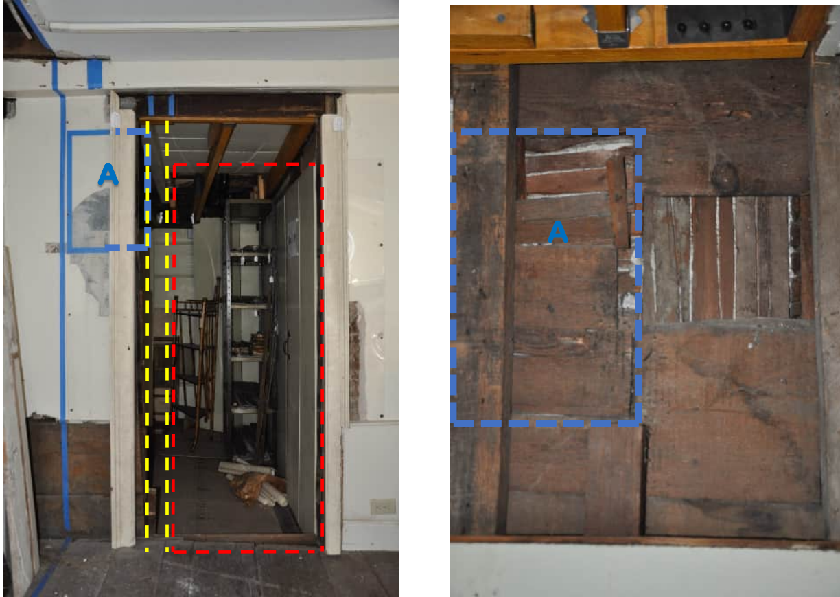
Figure 15. Left – View of the north wall of the hall (Rm 102), showing the current doorway to Rm 109 in the rear pile of the house. Throughout the 18 th century a smaller doorway opening provided access to the rear lean-to in this same location. Its approximate dimensions and location are indicated by the dashed red lines. The area within the blue rectangle A indicates the location of the former opening for a small wall cupboard or window opening. This opening was originally bounded on its east side by a wall stud which was later relocated several inches to the west when the doorway was enlarged. The yellow dashed lines indicate the original location of a Phase 1 wall stud which was relocated several inches to the west when the door opening was enlarged during Phase 4.
