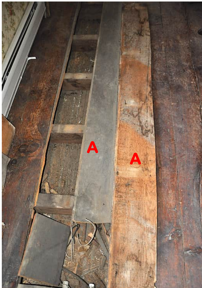
Figure 16. Removal of the Phase 2 floorboards and Phase 1 floorboard A in the floor of Rm 210 (over the parlor Rm 112) revealed absence of any discoloration on the joists and underside of the floorboard A due to smoke and soot. The ship-lapped Phase 1 flooring A was covered in Phase 2 in the early 19 th century with new square-edged pine boards. (Photograph by Myron O. Stachiw, 2024).
