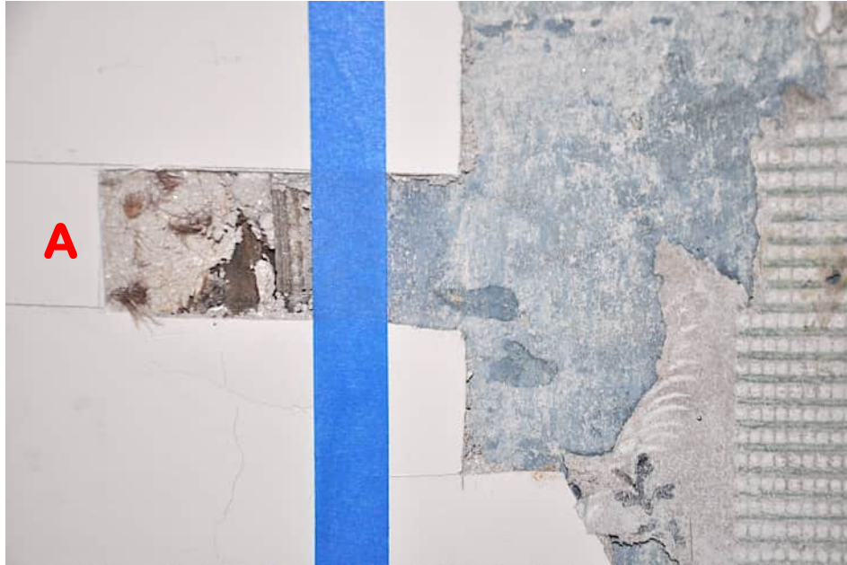
Figure 41. Detail view of the evidence of the former Phase 2 cupboard in Figure Y. The blue vertical line indicates the location of the east (front) face of the cupboard. A indicates an area where the Phase 4 plaster was applied to the north wall after the cupboard was removed. This plaster was applied over sawn- and split lath applied vertically, whereas the Phase 2 plaster (to the right of the blue line) was applied over horizontally-nailed lath. Note the blue paint and wallpaper to the right on the original Phase 2 wall finish, and the absence of blue paint on the plaster to the left of the blue vertical line. (Photograph by Myron O. Stachiw, 2024.)
