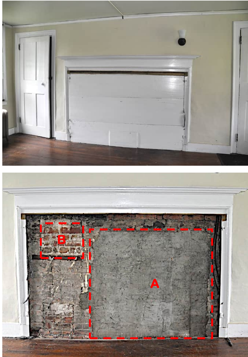
Figure 91. Two views of the rear ell kitchen fireplace in the north wall of Rm 107. The use of the fireplace A and bake oven B were discontinued during the second half of the 19 th century when a cast iron cook stove was installed. The fireplace- and bake oven openings were likely sealed with bricks and mortar during the 20 th century. Behind the doorway to the left of the fireplace is a small pantry with a pass-through opening in the north wall to Rm 107. (Photographs by Myron O. Stachiw, 2024.)
