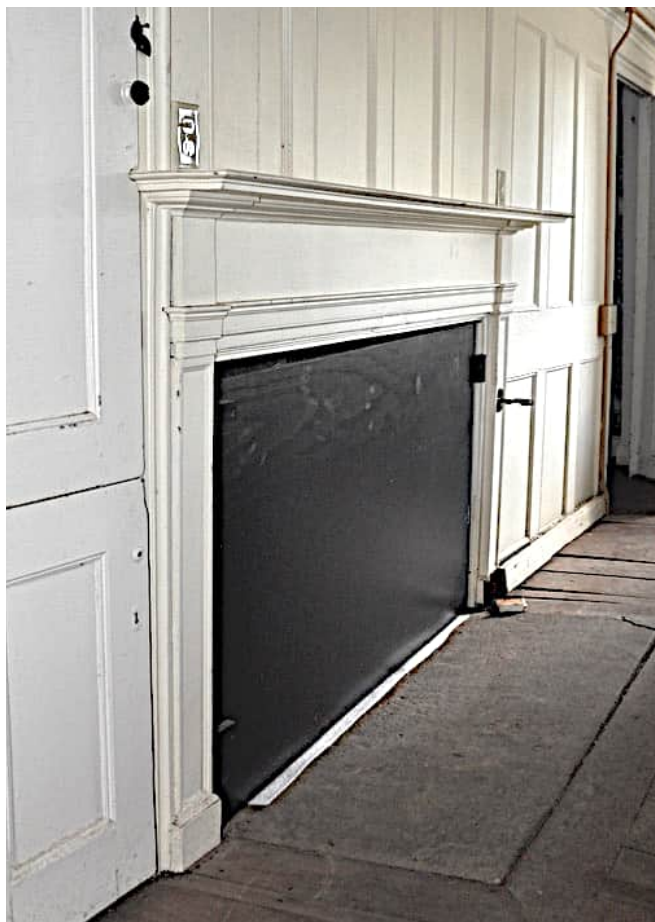
Figure 73 View of the Phase 4 mantelpiece applied to the east wall of the parlor (Rm 112). This mantelpiece replaced a Phase 3 fireplace surround composed of bold bolection molding (see Figures 48, 49). (Photograph by Myron O. Stachiw, 2024.)
