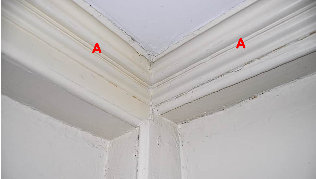
Figure 17. View of the casings applied to the posts and girts in the parlor (Rm 112) and the classically-inspired compound cyma recta and cyma reversa crown moldings applied over the girt- and summer beam casings. (Photograph by Myron O. Stachiw, 2024.)
