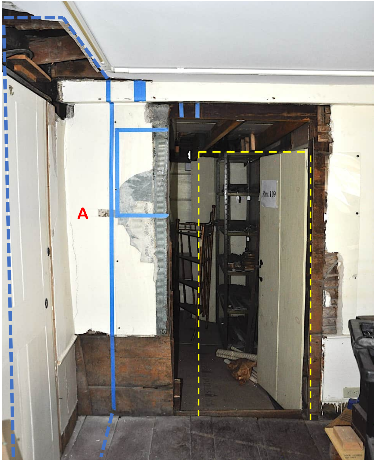
Figure 40. The dashed blue lines and the vertical blue line on the north wall of the hall/kitchen define the space occupied by the former Phase 2 cupboard. See Figure 41 for a detail view of the north wall at A . During Phases 1 and 2 the doorway from the hall/kitchen to the Phase 1- and Phase 2 rear lean-tos was smaller, as indicated by the yellow dashed lines. Enlargement of the doorway to its present size occurred during Phase 4. (Photograph by Myron O. Stachiw, 2024.)
