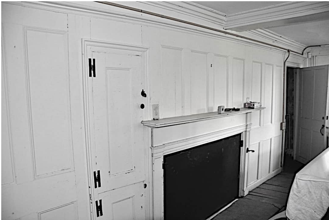
Figure 37. View of Phase 2 chimney breast wall paneling in the parlor (Rm 112). The flat panels and manner of construction of the paneled walls in both the hall/kitchen (Rm 102) and the parlor were identical. (Photograph by Myron O. Stachiw, 2025.)
