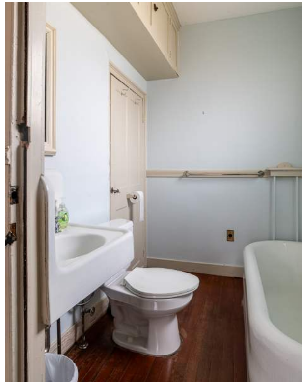
Figure 71. Shepherd House, east bathroom, second floor. Note early door at back left, re-set so that its superior face is oriented to the bathroom.
