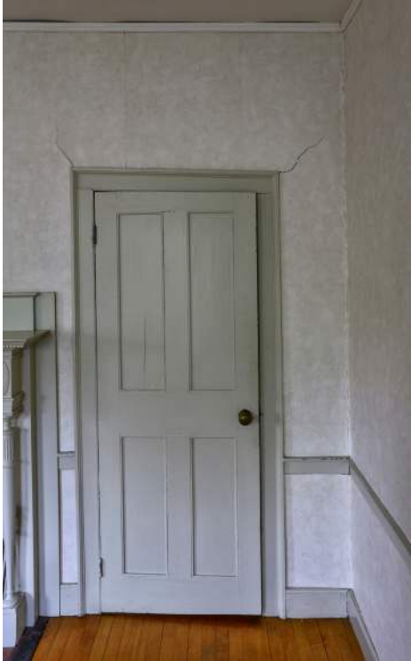
Figure 109. Room 210, Library Chamber, east closet door. Note how the top of the door opening slopes down on the right side towards the passage.
