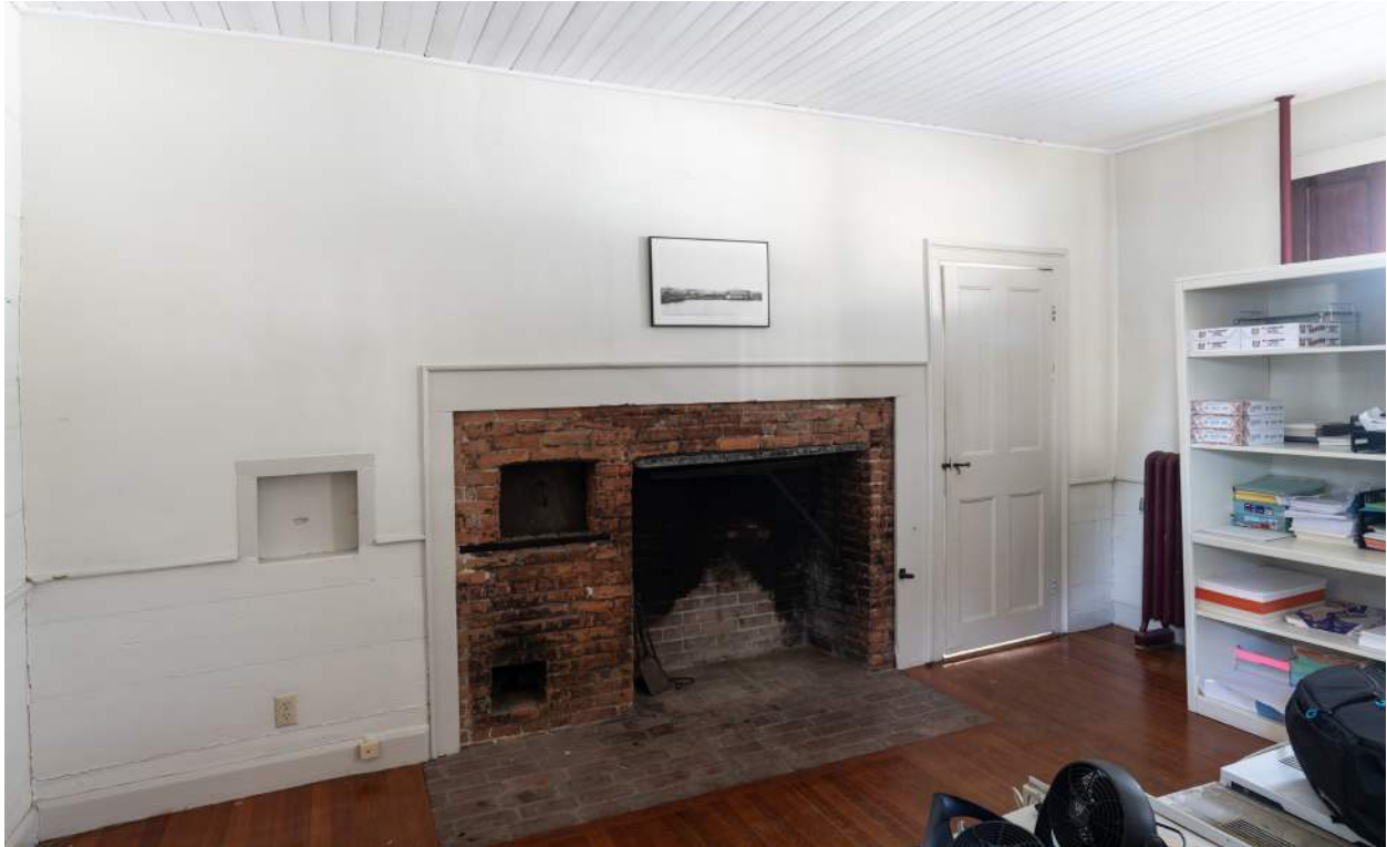
Figure 54. Shepherd House kitchen (room 105), view of fireplace wall. Note bake oven and sliding door to left of fireplace, providing access to dining room closet beyond..
