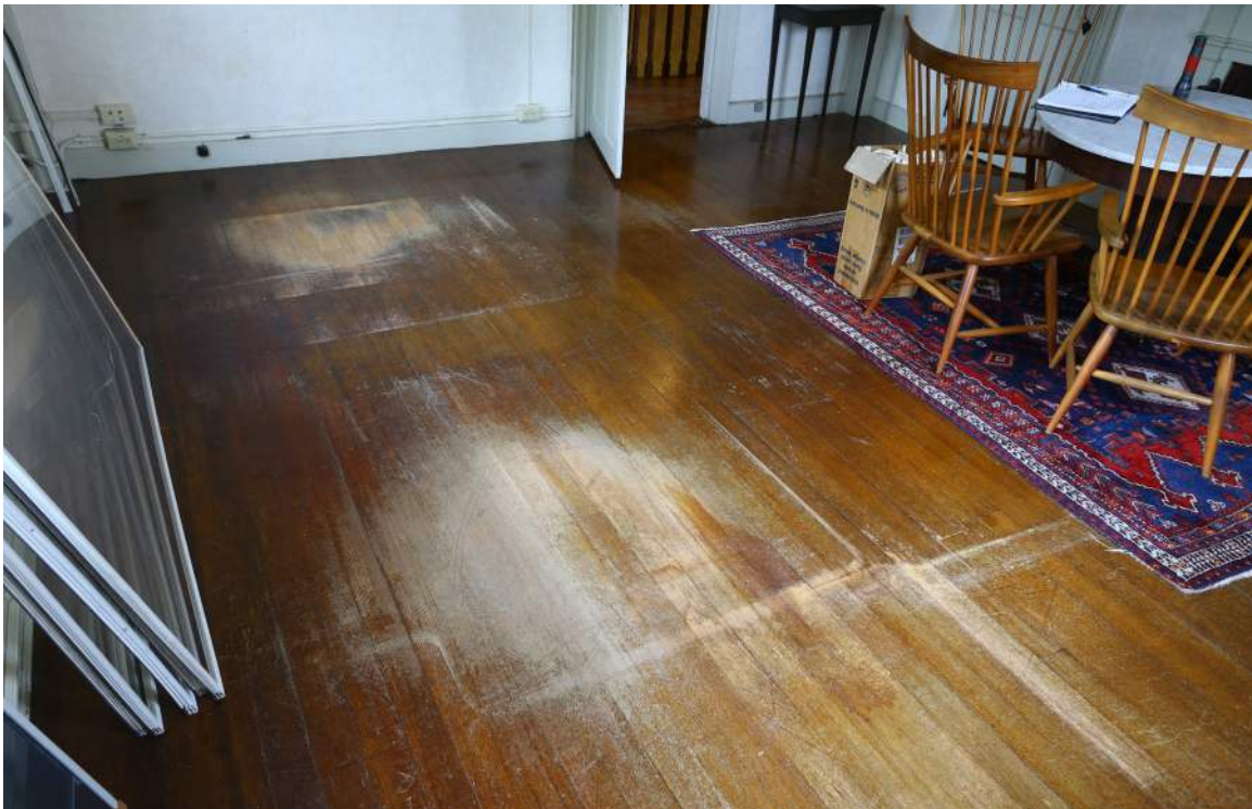
Figure 118. Flooring in Room 202. The floor finish is worn from years of desk chair use. Note surface mounted outlets on wall.
