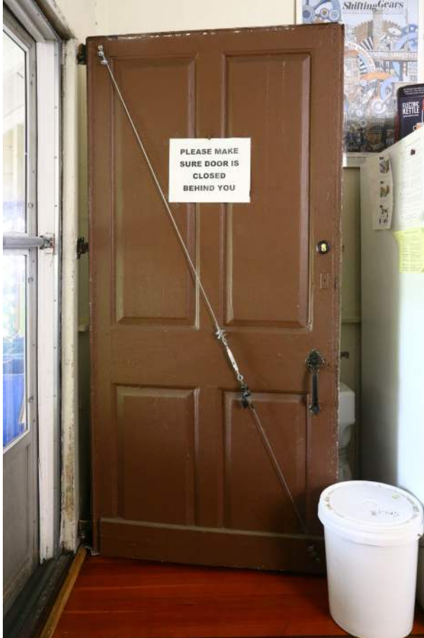
Figure 24. Shepherd House, detail of door to rear shed.
