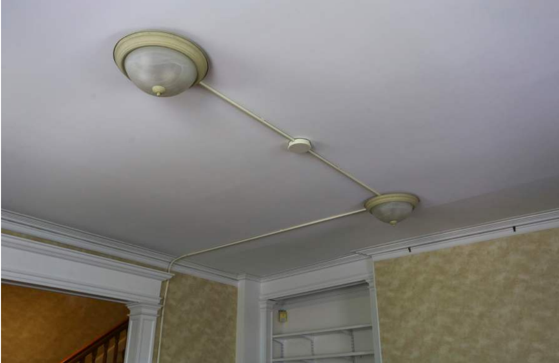
Figure 119. Example of modern light fixtures and surface mounted wire mold found throughout the house.
