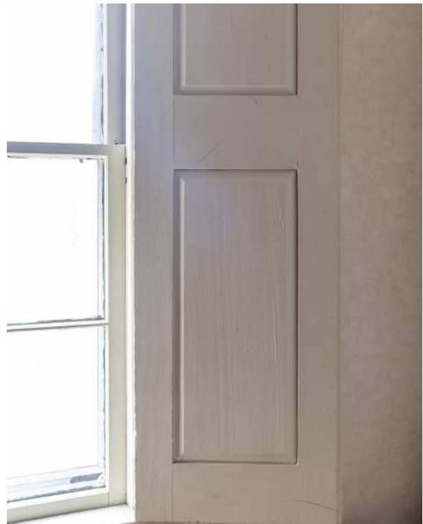
Figure 63. Shepherd House room over the entry (201), shutter detail.
