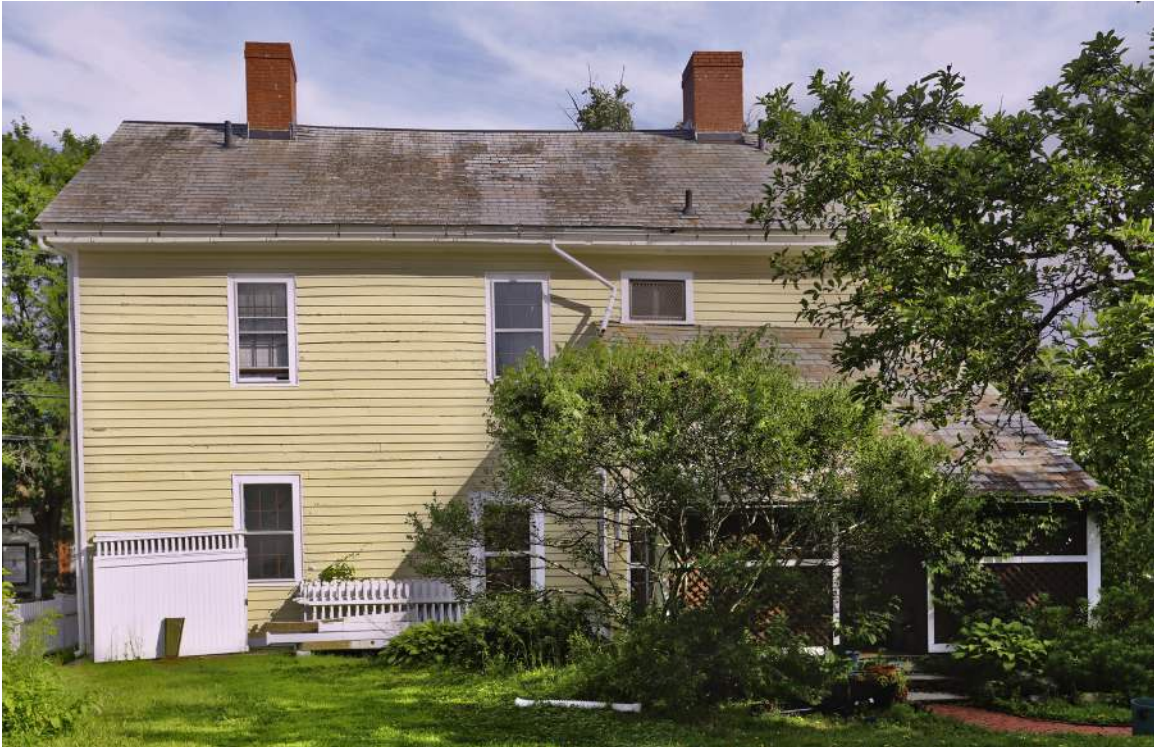
Figure 88. Shepherd House, north elevation. July 2024.
