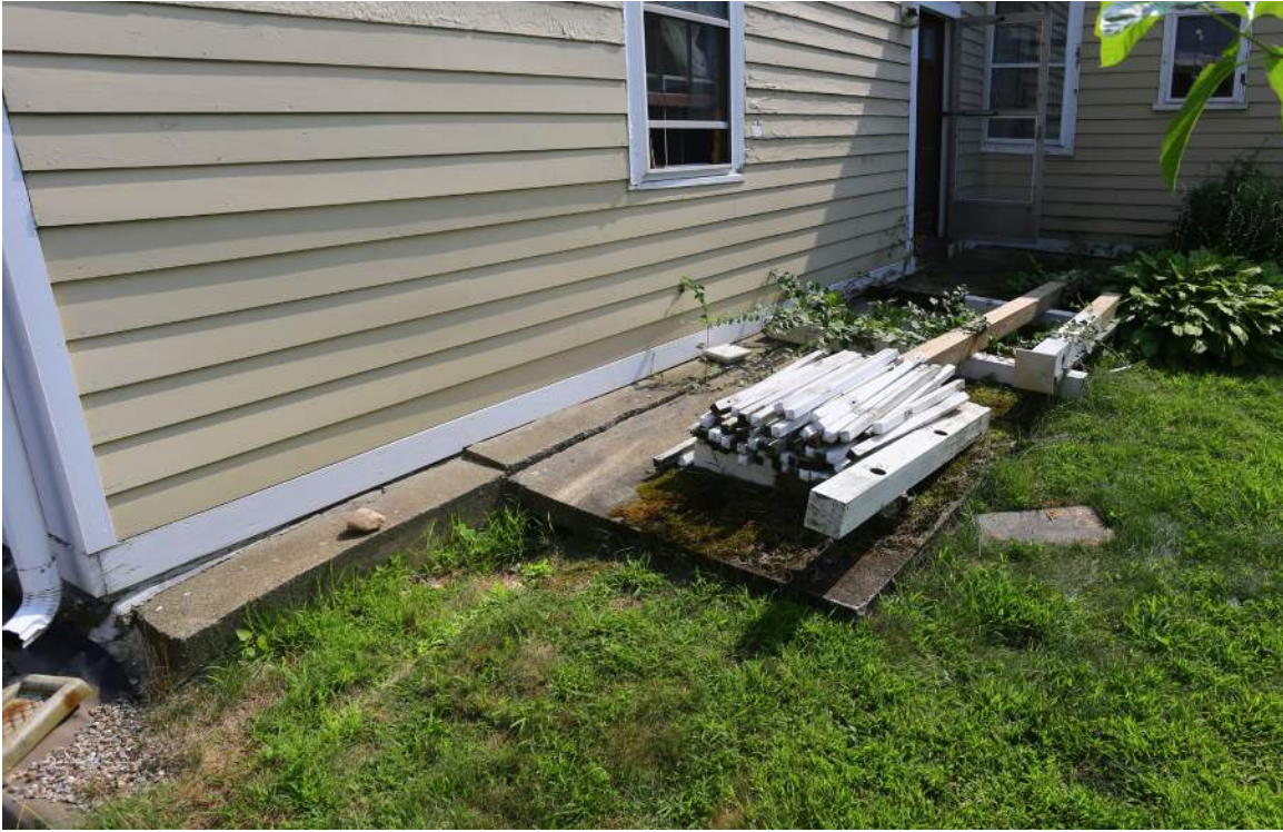
Figure 92. North elevation, east corner. The purpose and function of the concrete slabs and curbs poured against the foundation is not clear. They may be the remains of a patio area and/or to help buttress the stone foundation in this area. The concrete is unsightly and should be removed in combination with either regrading or improving the landscape in this area.
