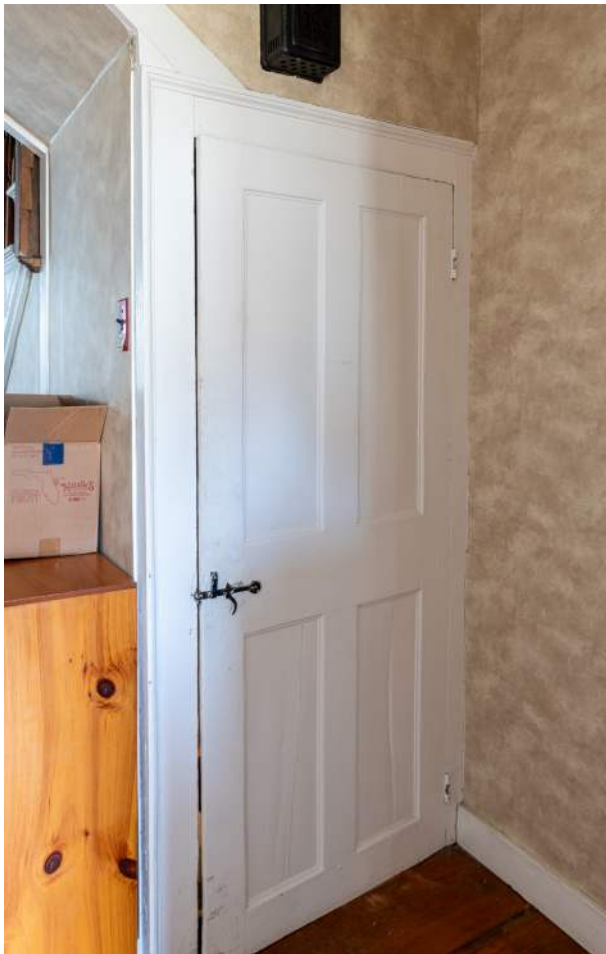
Figure 46. Shepherd House back passage, view of cellar stair door.
