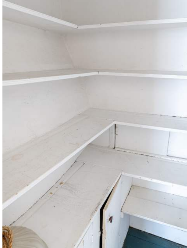
Figure 39. Shepherd House, dining room closet with early shelving and pass-through to kitchen, at lower right. Note plate rails.
