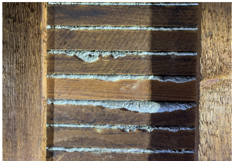
Figure 82. Shepherd House, attic, view of circular-sawn lath for room 302, visible in storage closet (room 303).
