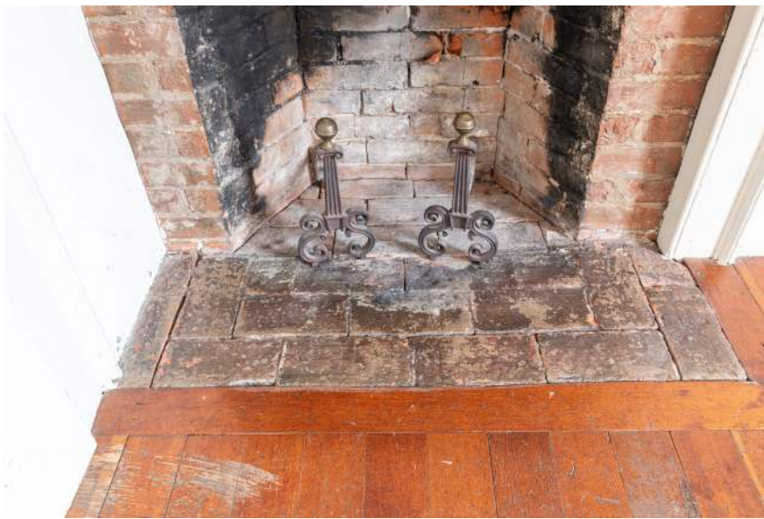
Figure 77. Shepherd House kitchen chamber, detail of firebox, hearth, and andirons. Note early flooring.
