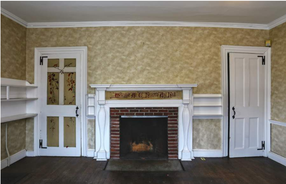
Figure 116. Room 109, former library. Early decorative paintwork from the Shepherd period has been preserved on the door and mantel, all other surfaces have received modern paint and wallpaper installed in c. 2007 when Mass Humanities occupied the building.
