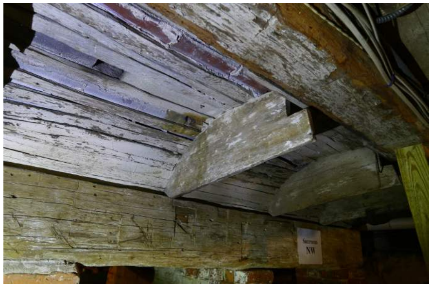
Figure 29. Shepherd House cellar, detail of hearth bed under kitchen (105).
