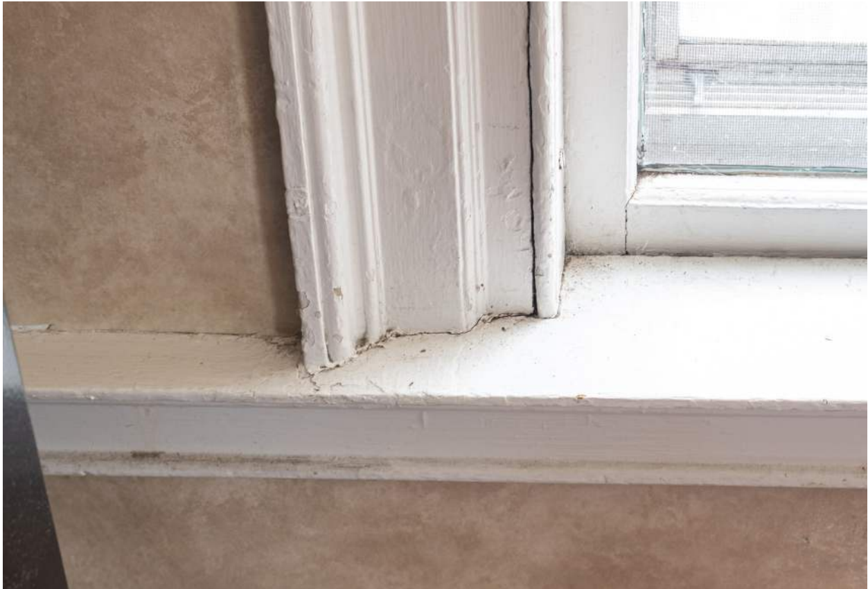
Figure 44. Shepherd House parlor (room 102), detail of window casing and sill.
