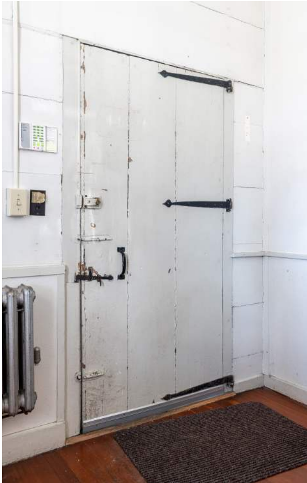
Figure 58. Shepherd House, service room (107) behind kitchen, detail of double-sheathed door to rear porch. Middle hinge modern.
