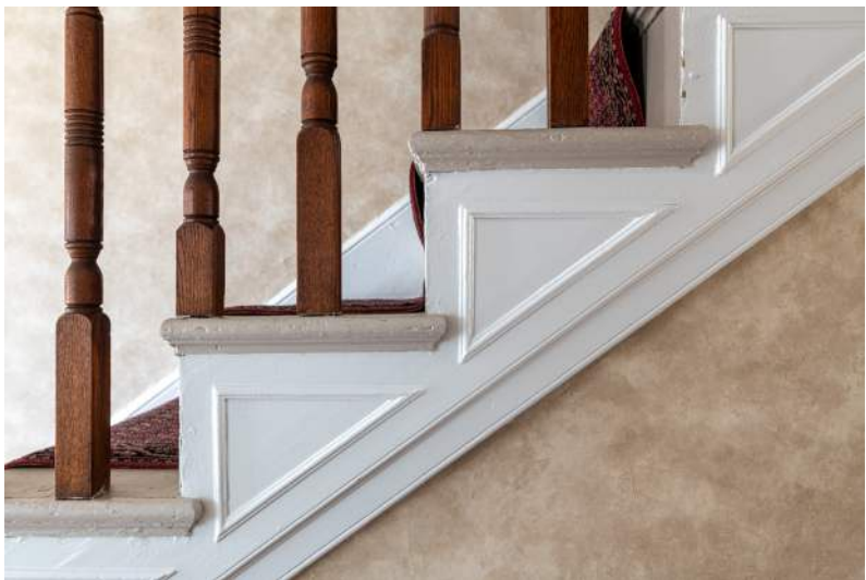
Figure 10. Shepherd House, front stair as altered c. 1900, detail of period IV baluster and period I applied bracket.
