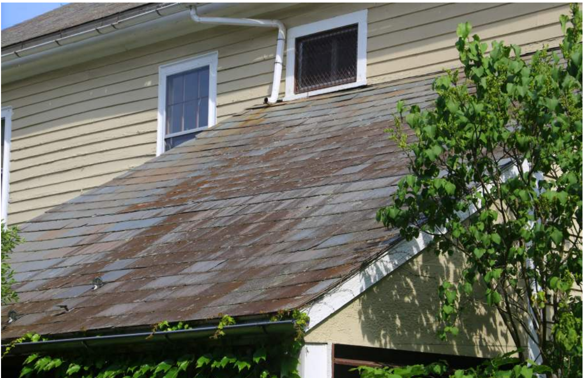
Figure 91. The slate roof on the lean-to is in good condition. A small amount of biological growth covers a portion of the slates. This can easily be removed using a mild detergent, light scrubbing and low pressure water.
