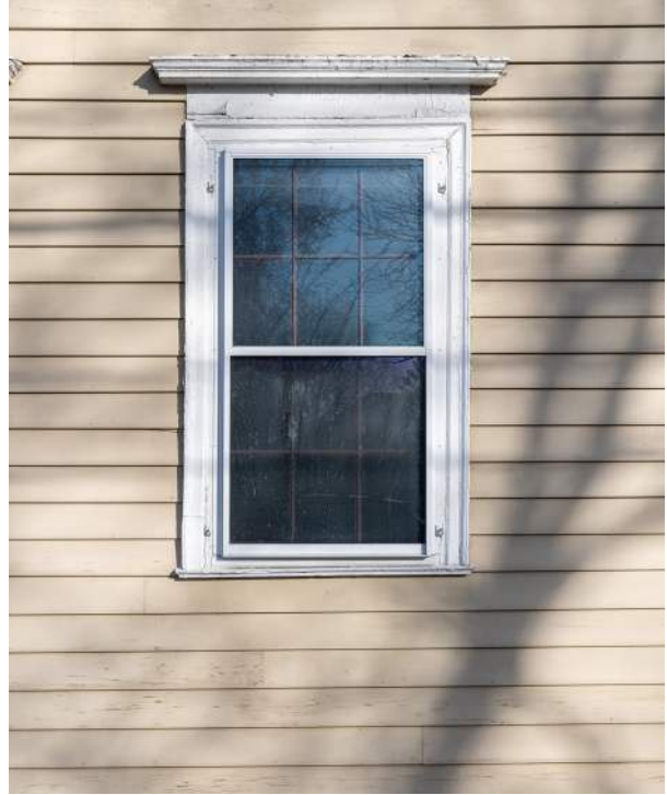
Figure 19. Shepherd House, detail of ground floor front window, east wall.
