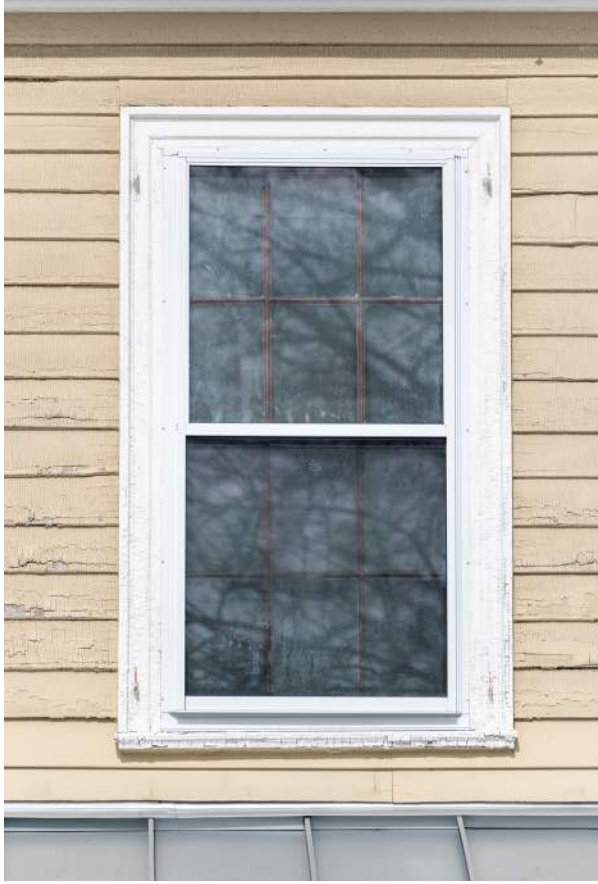
Figure 26. Shepherd House, period II second floor window, set in period I casing, in west wall.
