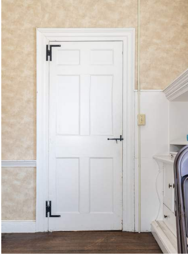
Figure 38. Shepherd House, dining room (room 100) door to passage. Thumb latch and H-L hinges installed mid-20th century.
