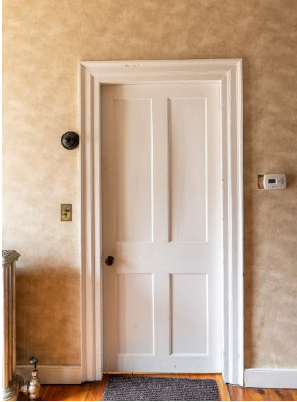
Figure 47. Shepherd House back passage, door to room 103.
