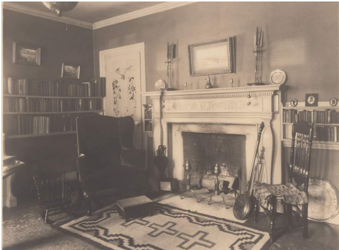
Figure 37. Shepherd House, c. 1924 photograph of dining room (room 100), following installation of shelving in 1902. Note replacement mantel, removal of patterned wallpaper, and installation of electrified ceiling light.
