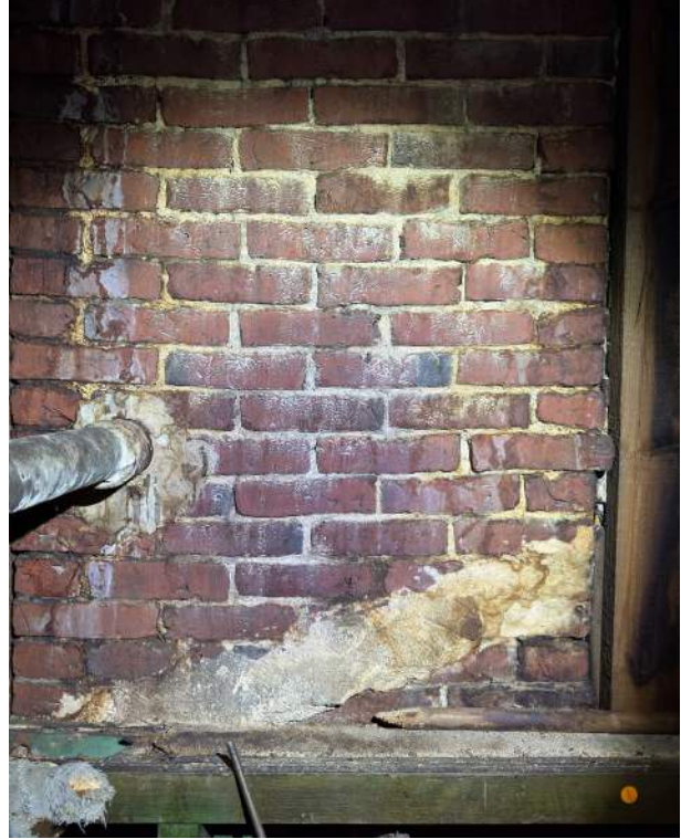
Figure 83. Shepherd House attic, view of rear of east chimney showing evidence for earlier roof in mortar flashing and projecting flashing course.
