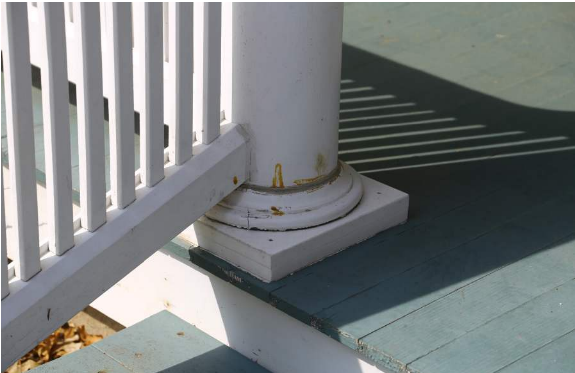
Figure 105. Detail of unpainted caulk/epoxy repairs to column base.
