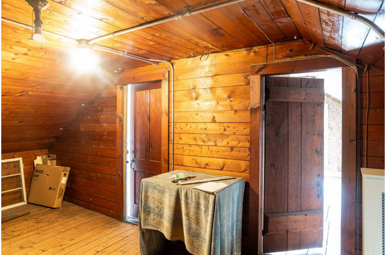
Figure 78. Shepherd House attic stair landing (301).
