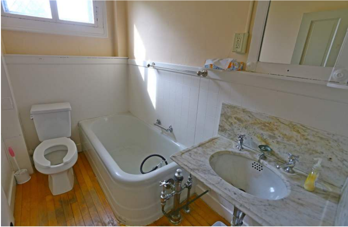
Figure 123. Room 206, bathroom. Representative example of early fixtures and plumbing remaining in the bathrooms. Water to the plumbing fixtures still remains active and the toilets and sinks are in use.
