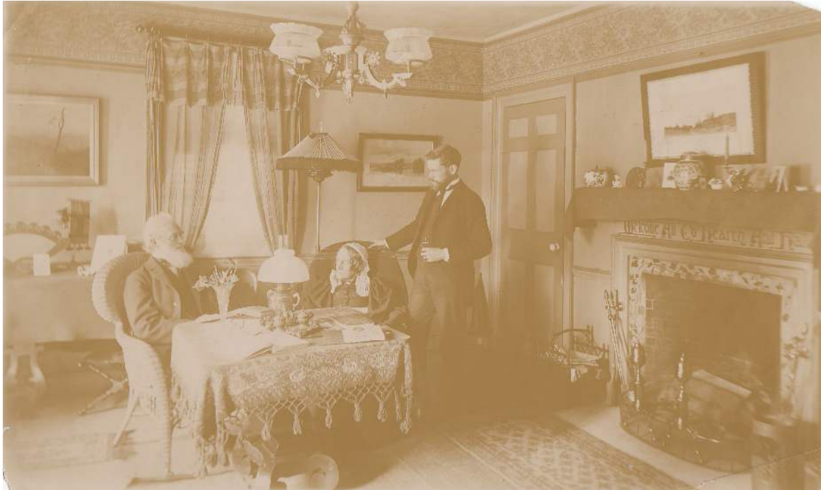
Figure 36. Shepherd House, photograph of Shepherd family in room 100 taken c. 1896. Note original mantel still in place; molded surbase with no shelving or built-in seating, wallpaper border, and ceiling light fixture. Photograph courtesy of Historic Northampton.
