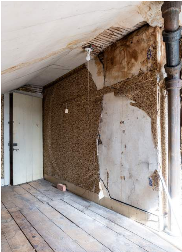
Figure 84. Shepherd House rear attic chamber (304) with circular-sawn lath in ceiling and cast iron plumbing vent pipe.
