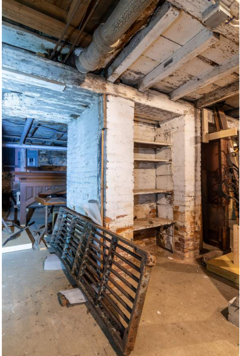
Figure 28. Shepherd House cellar, showing base for east chimney.
