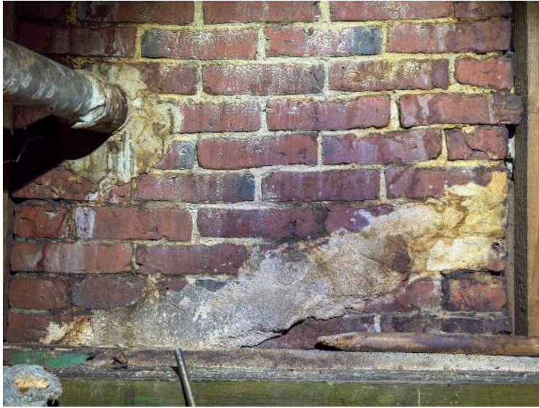
Figure 8. Shepherd House attic, view of rear of east chimney showing evidence for earlier roof in mortar flashing and projecting flashing course.
