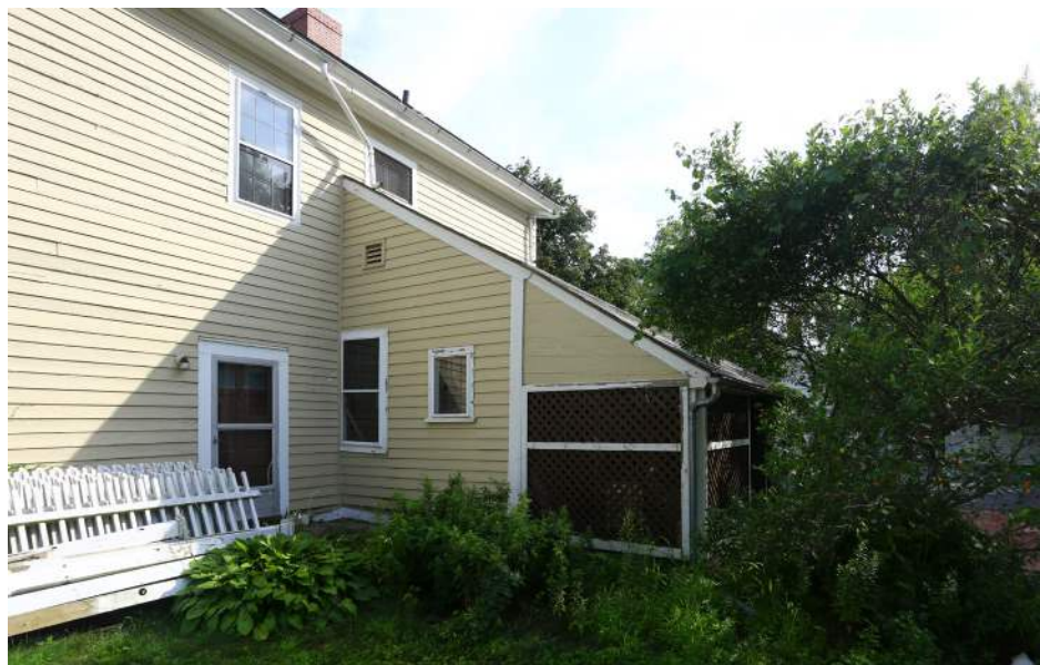
Figure 23. Shepherd house, view of rear shed and enclosed porch.
