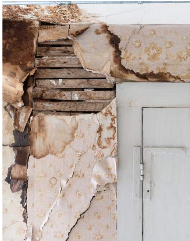
Figure 81. Shepherd House, attic chamber (305), detail of cut-nailed, circular-sawn lath and H-L hinge secured with flat-head screws.
