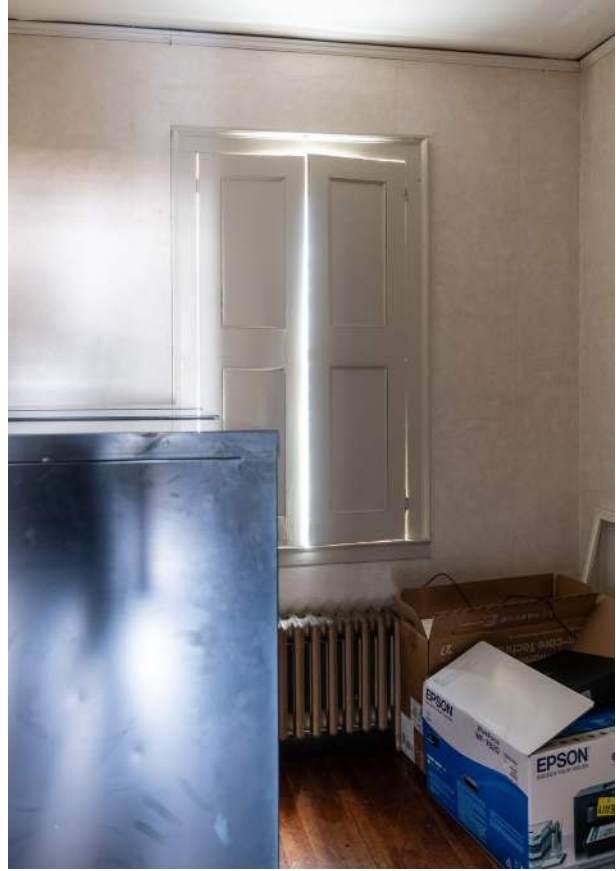
Figure 62. Shepherd House, room over the entry (201).
