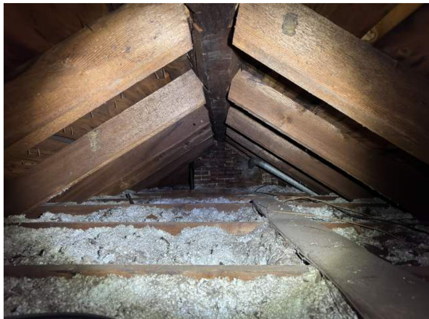
Figure 79. Shepherd House attic, view of rafters and ridge beam.
