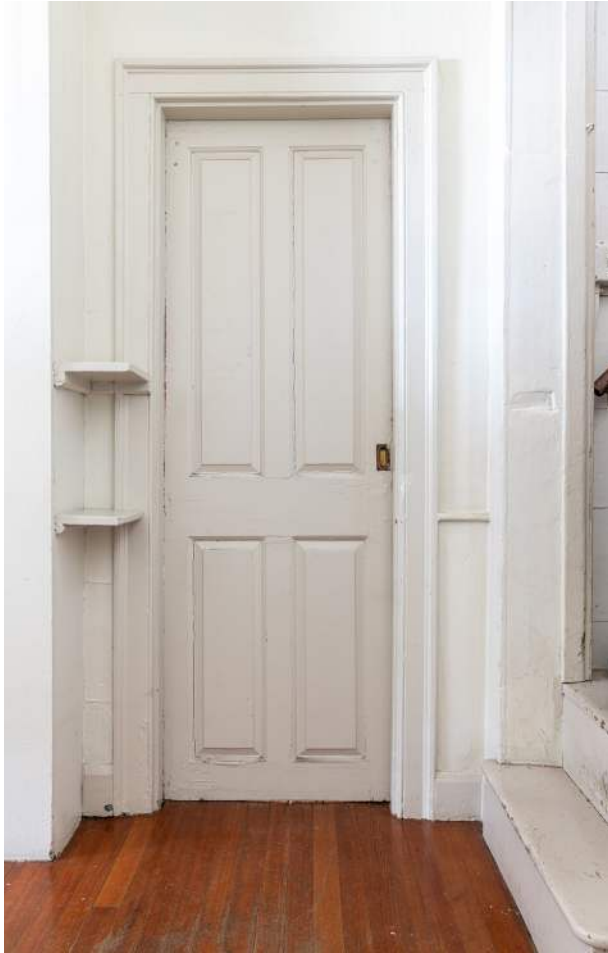
Figure 56. Shepherd House kitchen door to pantry (107), originally hung on H-L hinges, reset as pocket door c. 1900.
