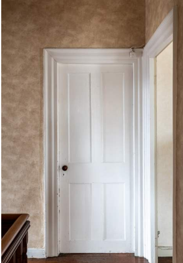
Figure 61. Shepherd House, second floor passage, door to parlor chamber (202).
