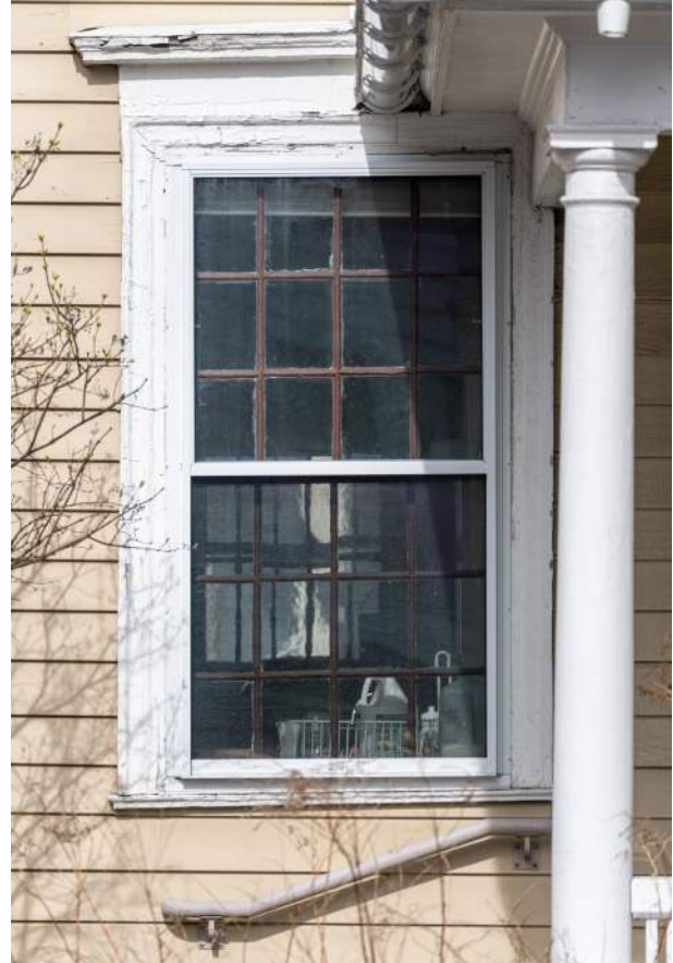
Figure 27. Shepherd House, period I ground floor window in service room behind kitchen. Note 12-over-12 sash.
