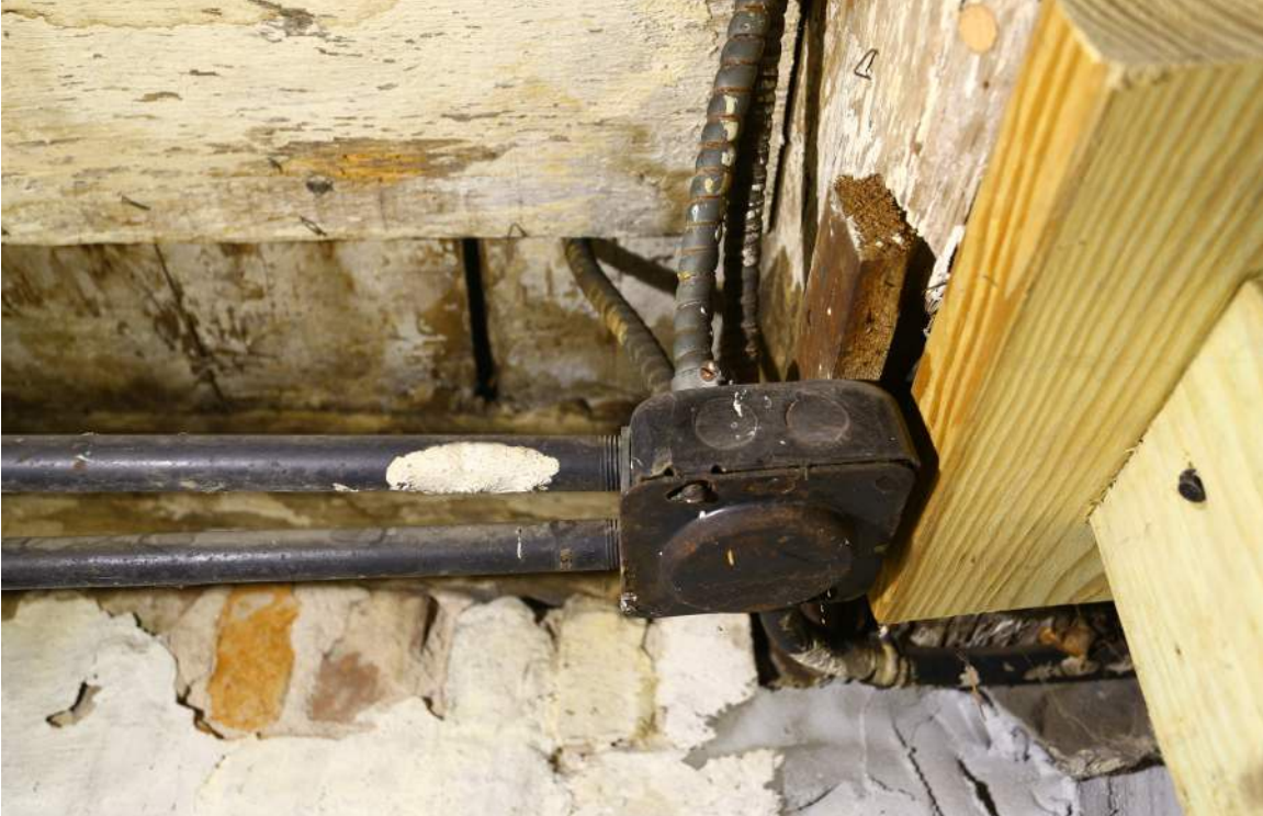
Figure 129. Much of the early 20th century electrical service remains in place and active. In the cellar, this takes the form of cloth covered wiring run in conduit and BX (flexible metal cable) run up into the wall cavities. This wiring likely dates to the second quarter of the twentieth century when the house was wired for electricity.
