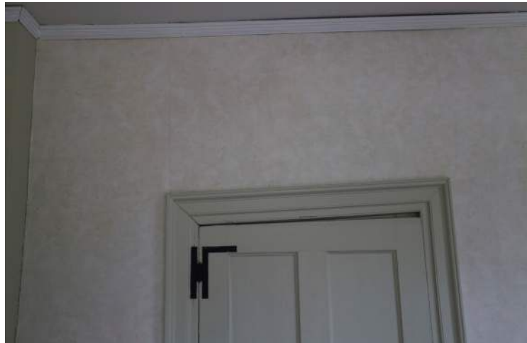
Figure 112. Detail of the top of the closet door opening in previous photo.
