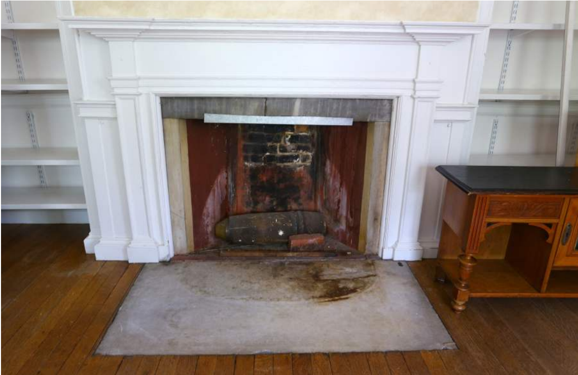
Figure 121. Representative example of the metal flange for the flue closures found at the fireplace openings. The profile of the stain on the hearth together with the ghosts on the jambs of the fireplace suggest a stove of some sorts may have once been located here. The stain on the hearth should be gently cleaned to remove surface soiling.
