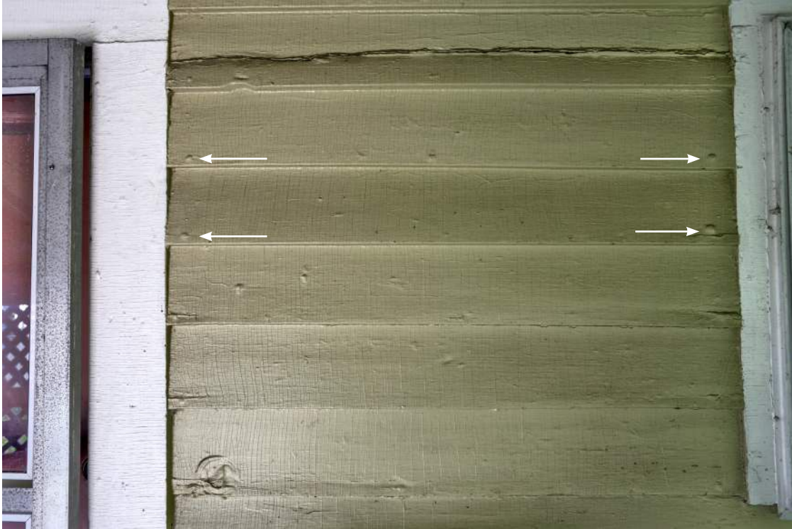
Figure 94. Original clapboards on the north elevation within the lean-to. Arrows point to the painted over heads of wrought nails used to fasten the clapboards to the building.
