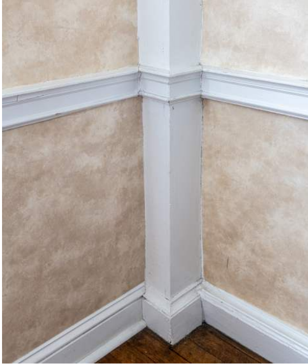
Figure 43. Shepherd House parlor (room 102), detail of southwest corner post with early dado cap.
