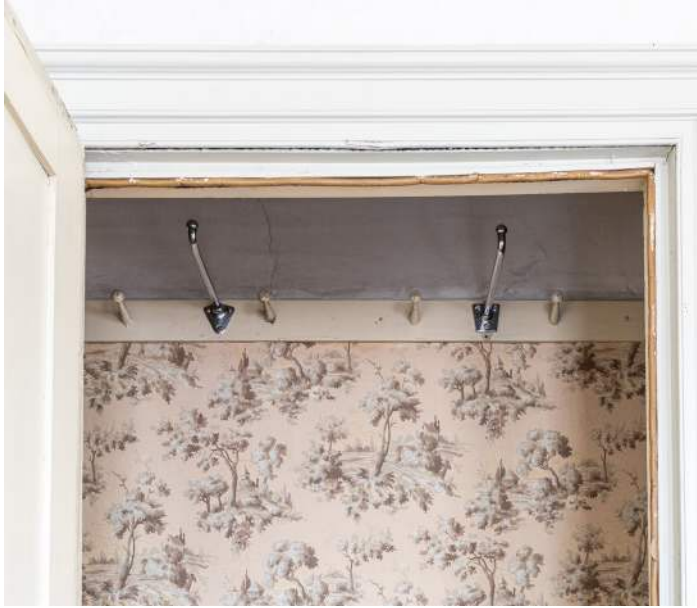
Figure 70. Shepherd House parlor chamber closet with early peg rail.
